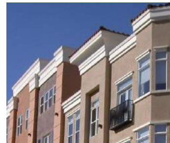
Variety in building height
