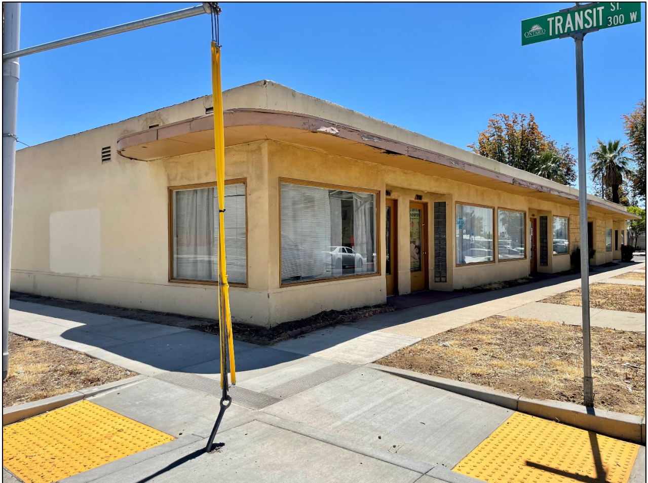
Office Building- 201-215 S. Fern Avenue
