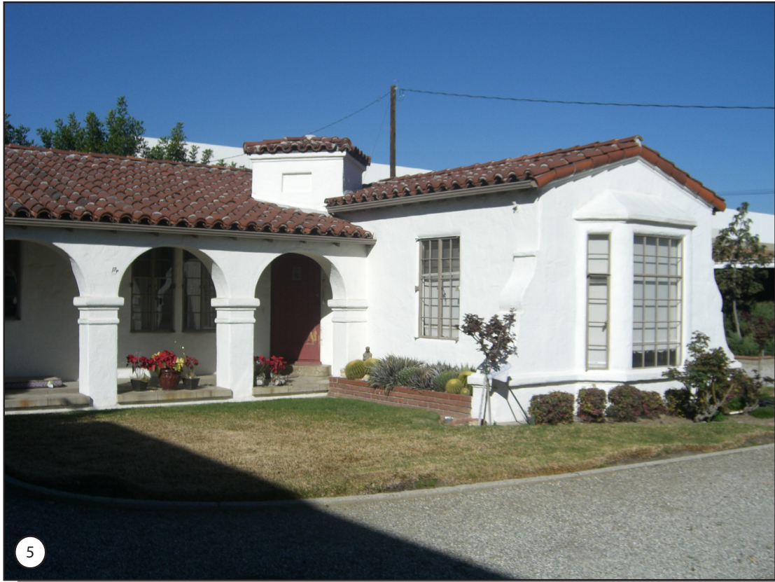
Photograph 5: Residential House, View towards the west.
