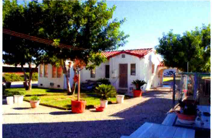
West and south elevation, view northeast
