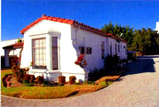
North elevation (and partial east elevation), view southwest
