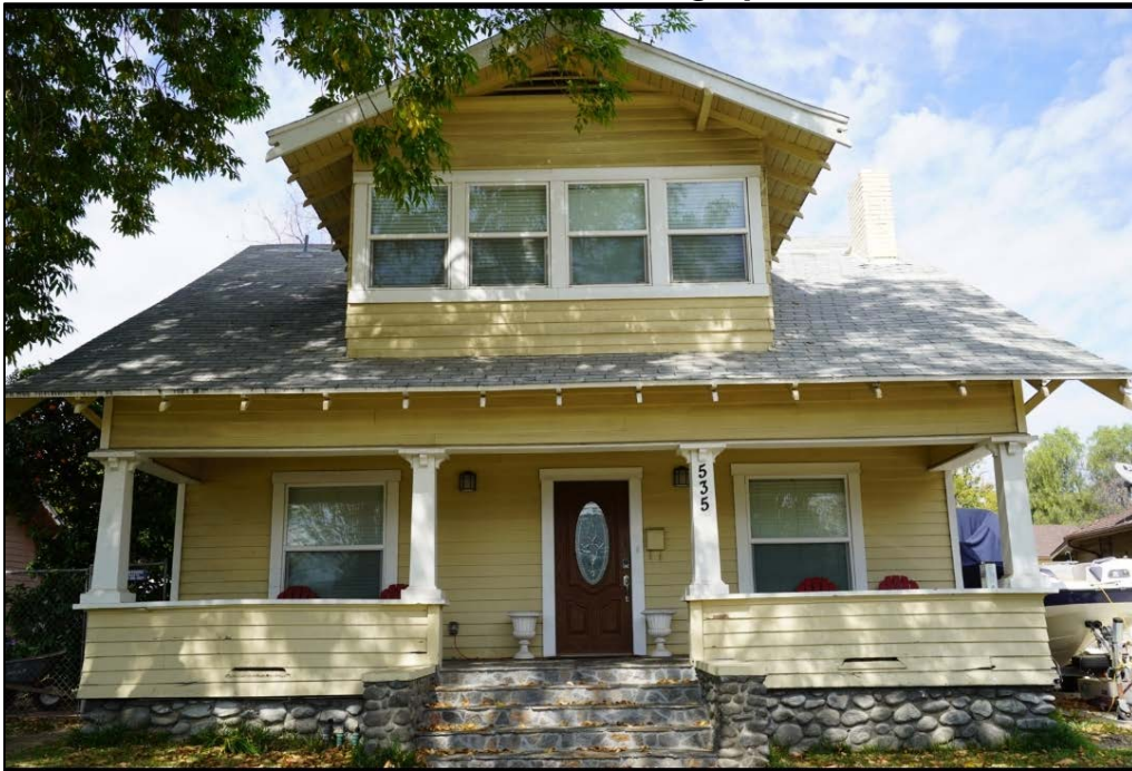
Primary Façade (south elevation)
