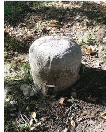
Image 24. View of the water standpipe (Resource No. 17).
