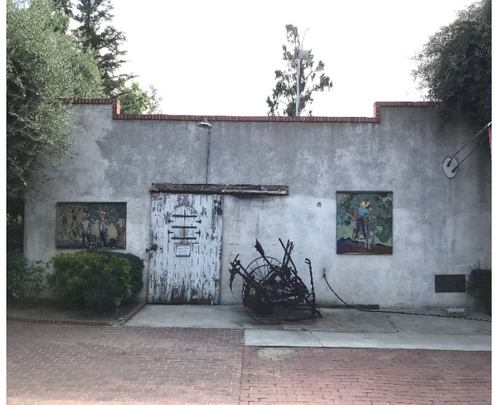
Image 2. View of west elevation of the Vat, Grading, Filling, Canning, and Museum Rooms building (Barn 2) depicting the murals next to the museum entrance (Resource No. 2). This building is a portion of the Olive Canning Processing Facility.
