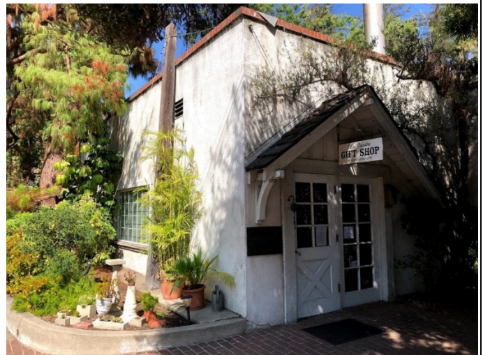
Image 12. View of the southwest corner of La Casita Gift Shop building (Resource No. 4).
