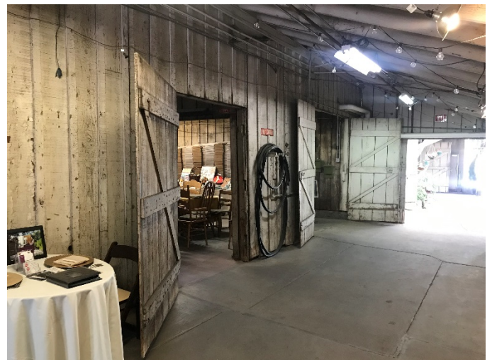
Image 8. View of south façade of the Original Barn, Olive Sheds, Boiler, and Labeling Rooms building (Resource No. 5). Other portion of the Olive Canning Processing Facility.
