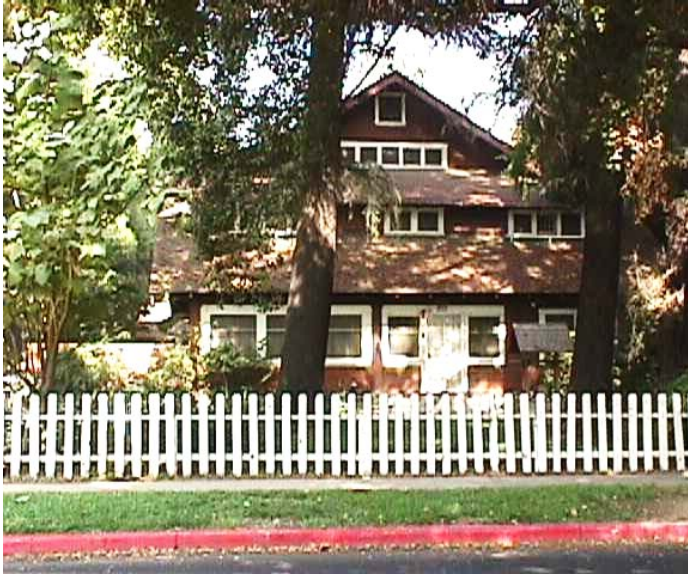
Image 1. View of south elevation of the Clifford C. Graber House (Resource No. 1).
