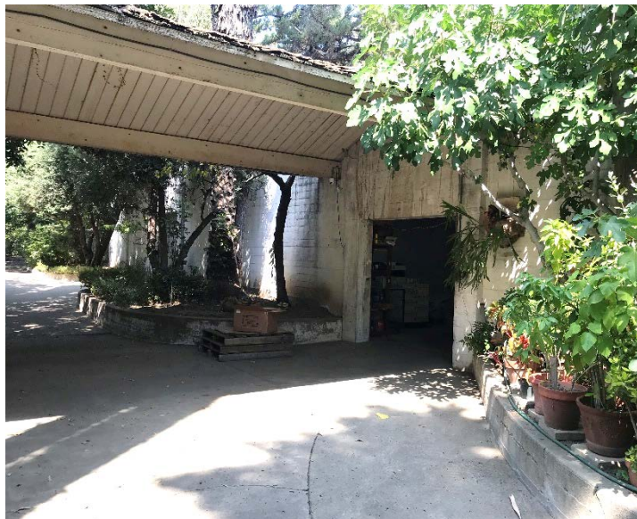
Image 14. View of west elevation of Warehouse A building (Resource No. 7) showing breezeway connection.
