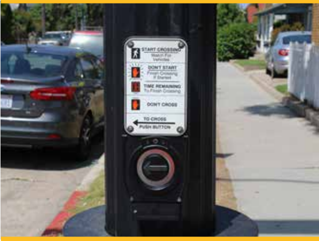
Accessible Pedestrian Signal
