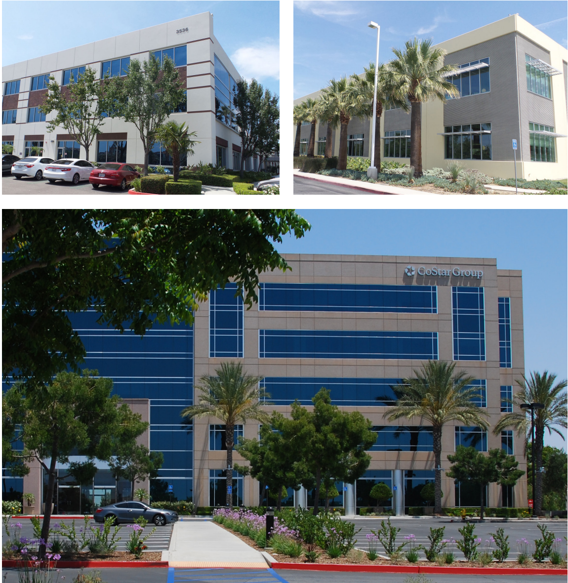
Figure 3.3: Photographs of Existing Office Buildings in the OCSP
