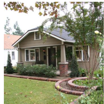
Tapered posts with brick bases, grouped windows and wood detailing.
