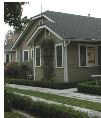
Wrap material, gable end treatment and window detailing to side elevation where required.
