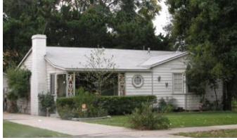
Long horizontal gable roof, with extensive use of lap siding and brick accent at chimney.
