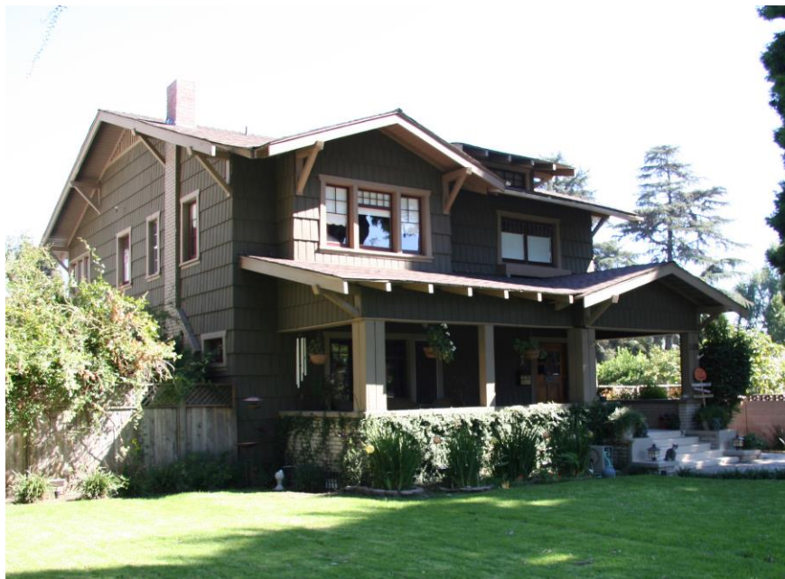
Articulated and asymmetrical two-story massing, extensive shingle siding, large porch, and appropriate geometry for divided lights and multi-paned glass.
