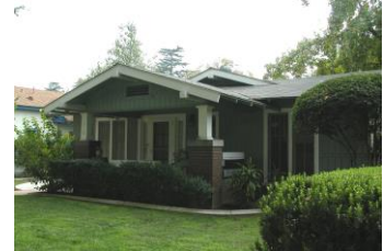
Entry door with side lights, shingle siding and wood posts with brick bases.
