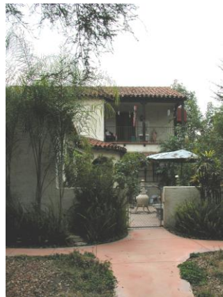
Heavy timber Deck Overlooking Entry Courtyard below
