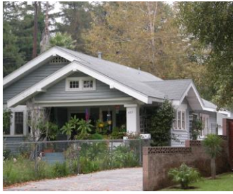
Low slope gabled roofs with large overhangs.
