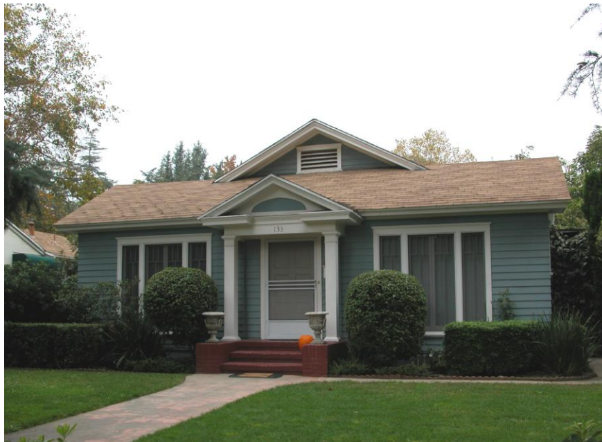
One story massing with windows grouped to mimic French doors with side lights, gable end treated with vent.
