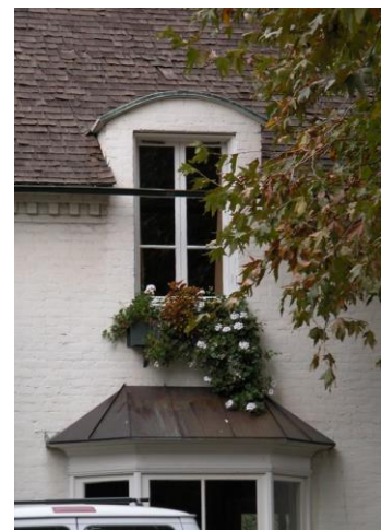
Use of multi-paned dormer and bay windows.
