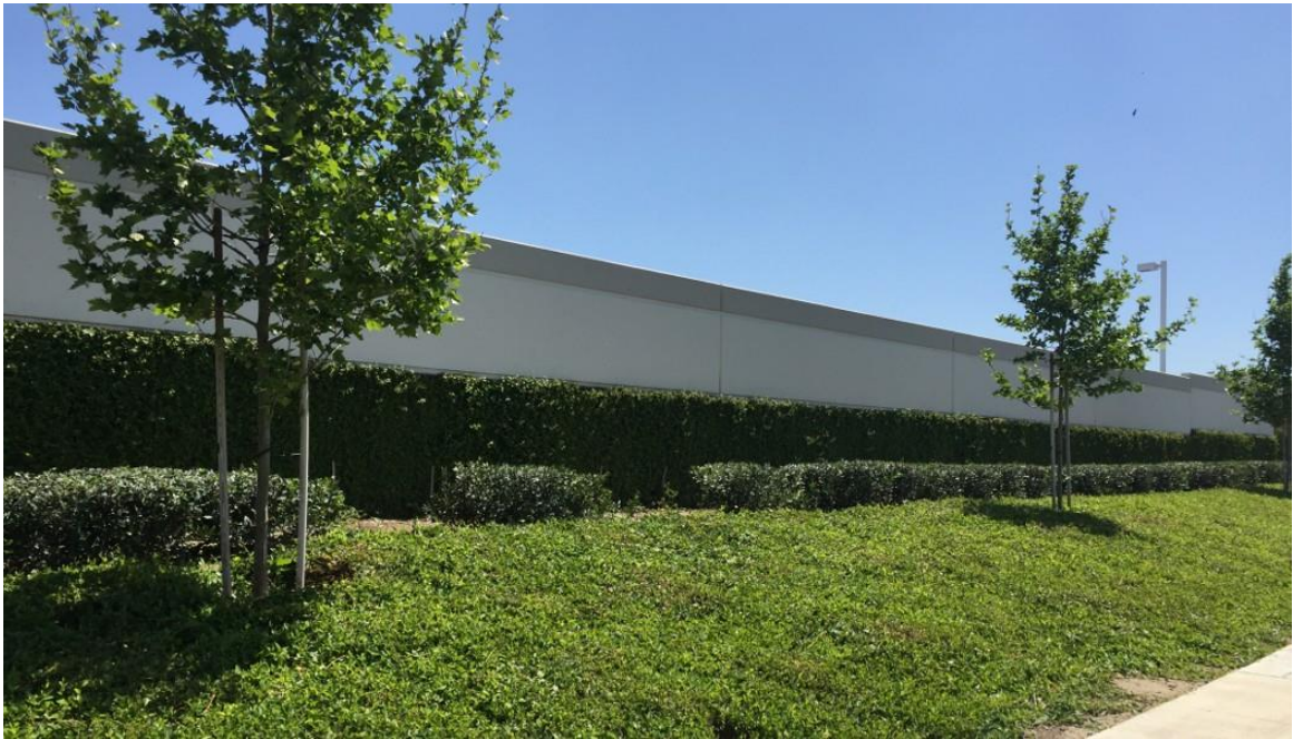
Photo 7.4-Example of typical screen wall with landscaping
