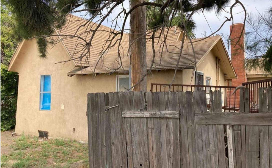
Photograph 2: 14095 Euclid Avenue, south elevation, camera facing north, May 22, 2023.
