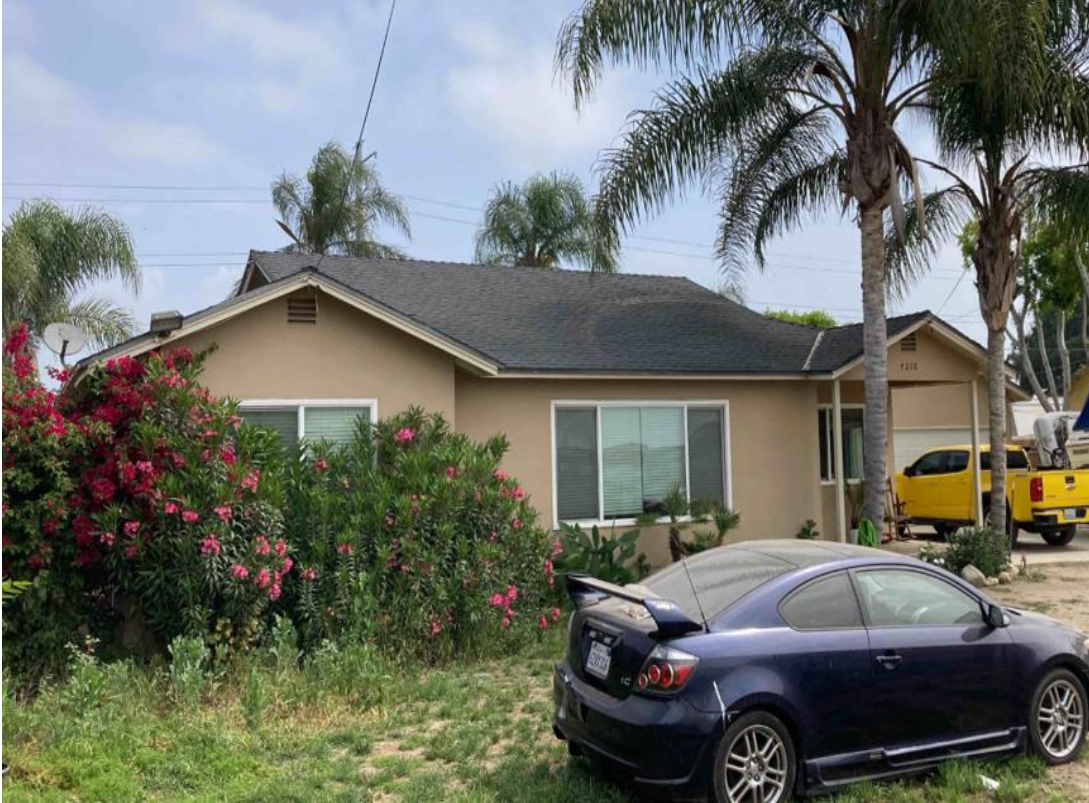
Photograph 2: 7218 Edison Avenue, south elevation, camera facing northeast, May 22, 2023.
