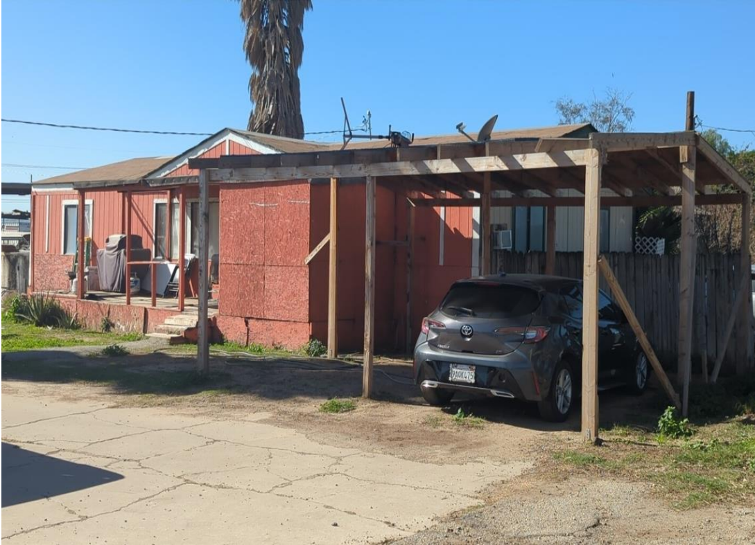
Photograph 9: Residence east of residential/storage building, east elevation, camera facing southwest, February 8, 2023.
