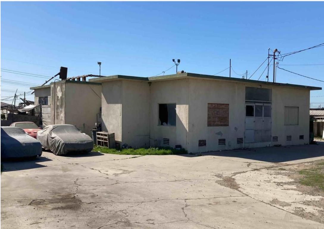
Photograph 10: Eastern Milk Parlor, east and north elevations, camera facing southwest, February 8, 2023.
