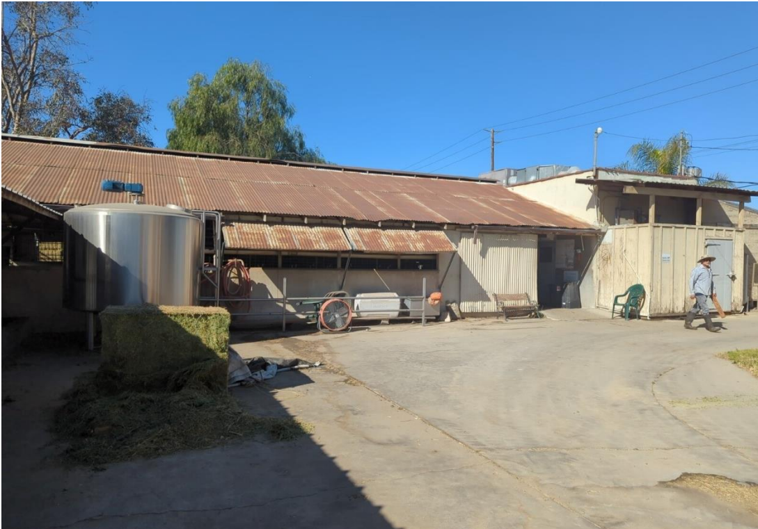
Photograph 4: Western milking parlor, rear section left frame, east elevation, camera facing southwest, February 8, 2023.
