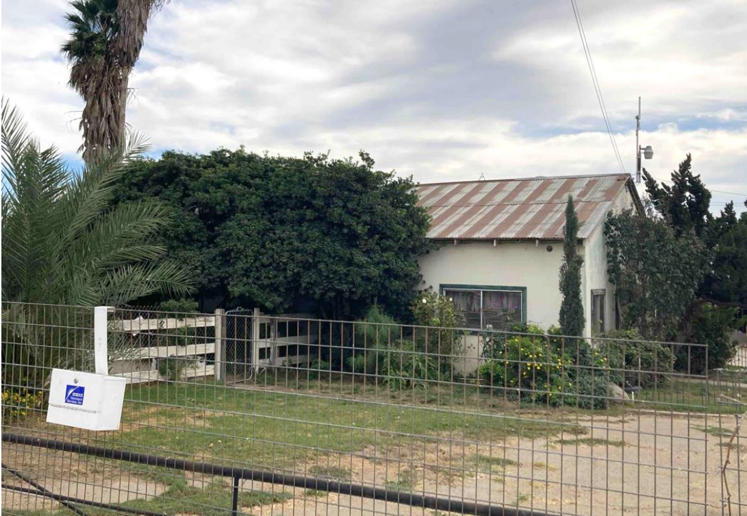
Photograph 7: Residence/storage building, north and west elevations, camera facing southeast, October 31, 2022.
