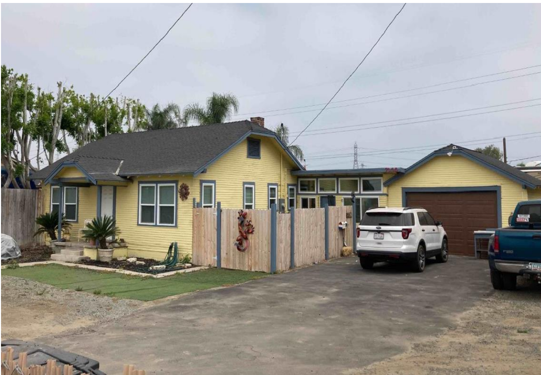
Photograph 3: 7226 Edison Avenue, south and east elevations, camera facing northwest, May 22, 2023.
