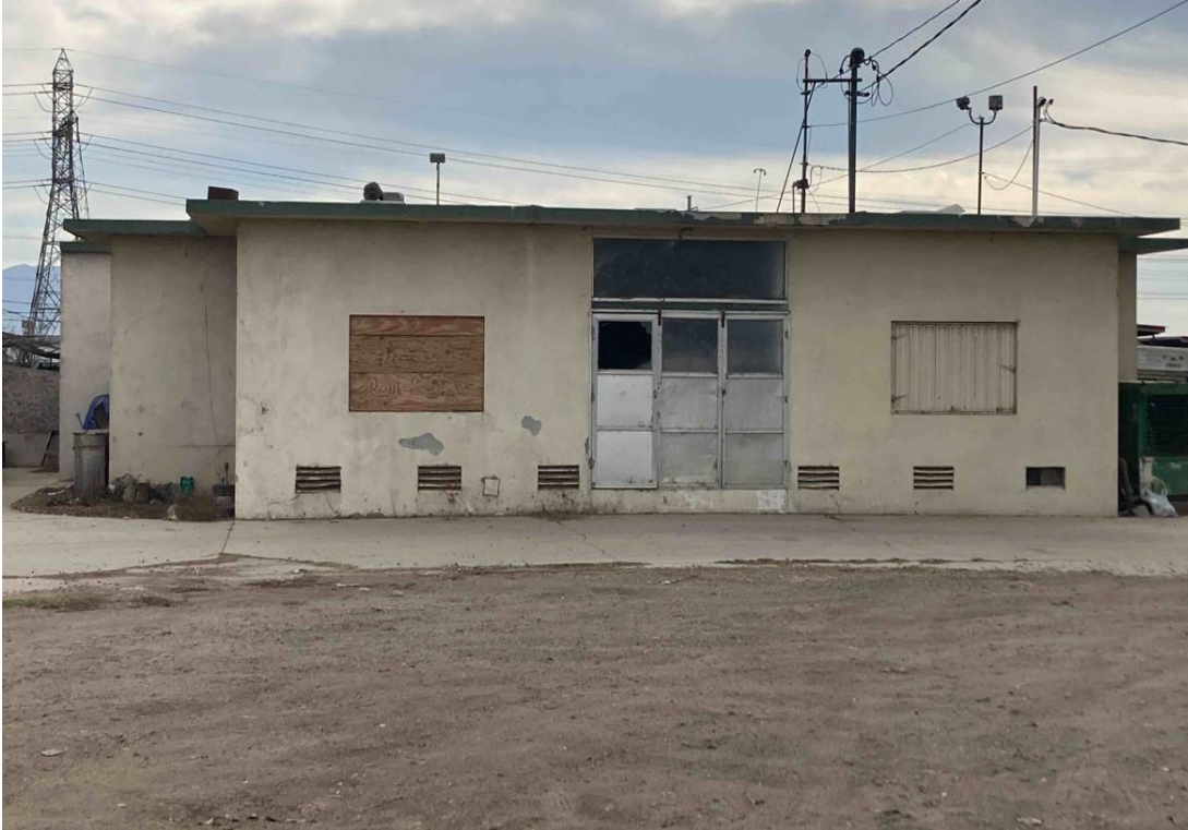
Photograph 11: Eastern Milk Parlor, north elevation, camera facing south, February 8, 2023.
