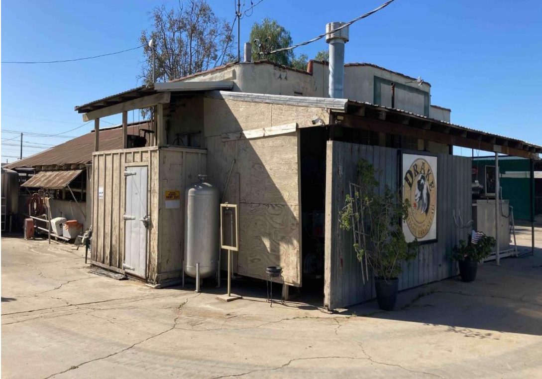
Photograph 3: Western milking parlor, east and north elevations, camera facing southwest, February 8, 2023.
