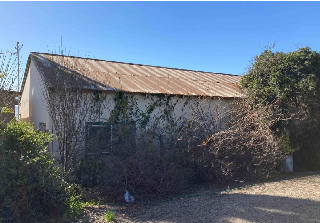
Photograph 6: Residence/storage building, east and north elevations, camera facing southwest, February 8, 2023.
