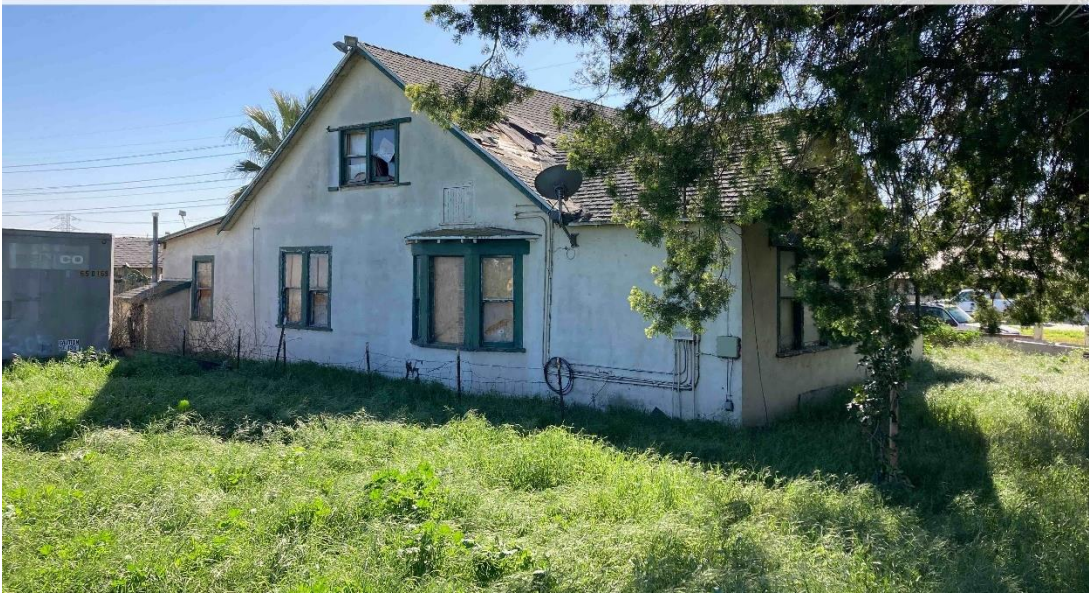
Photograph 2: 13813 Euclid Ave residence, east and north elevations, camera facing southwest, February 8 2023.
