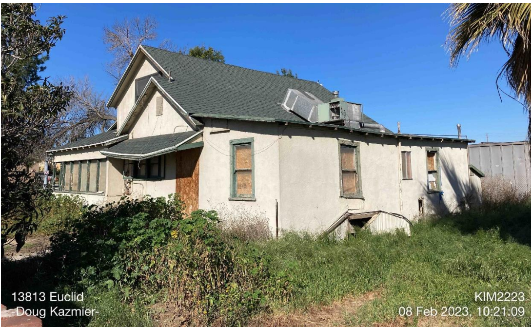
Photograph 3: 13813 Euclid Ave residence, west and south elevations, camera facing northeast, February 8, 2023.
