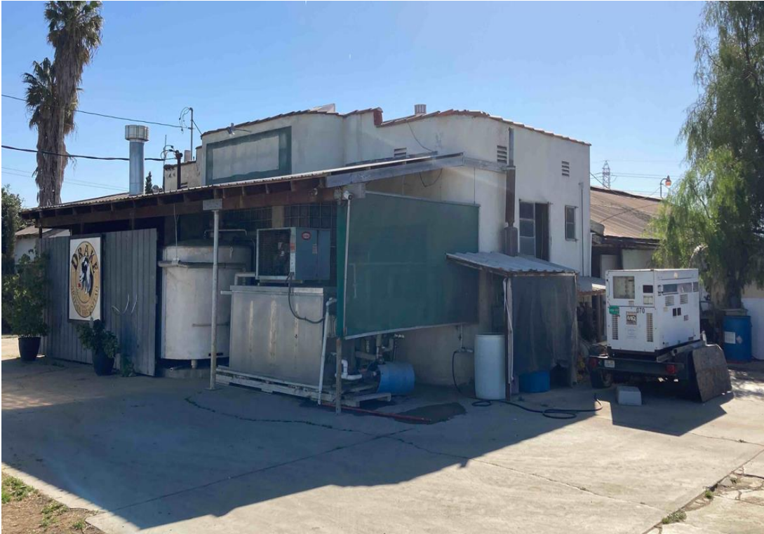
Photograph 2: Western milking parlor, north and west elevations, camera facing southeast, February 8, 2023.
