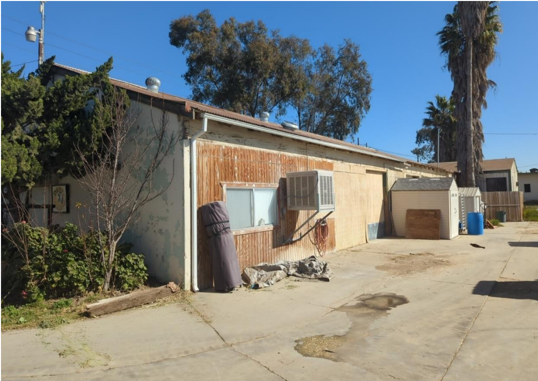
Photograph 8: Residence/storage building, west and south elevations, camera facing northeast, February 8, 2023.
