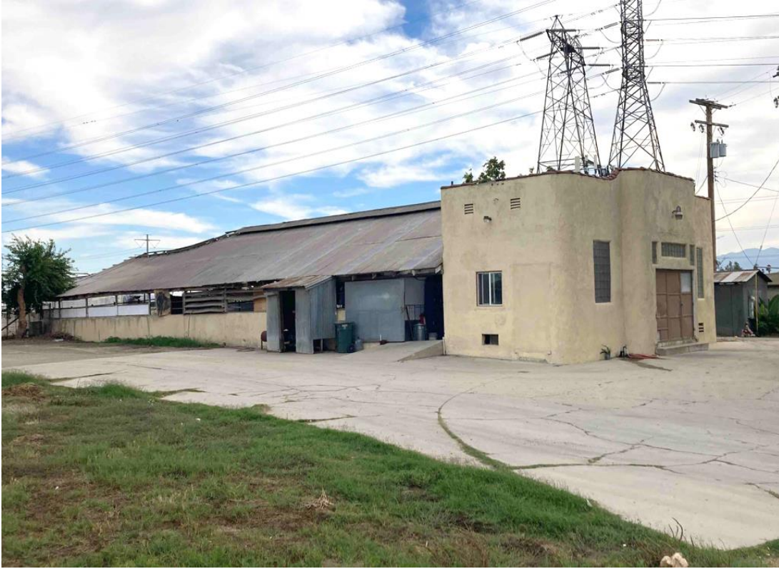
Photograph 6: 13813 Euclid Ave milk parlor, north and west elevations, camera facing southeast October 31, 2022.
