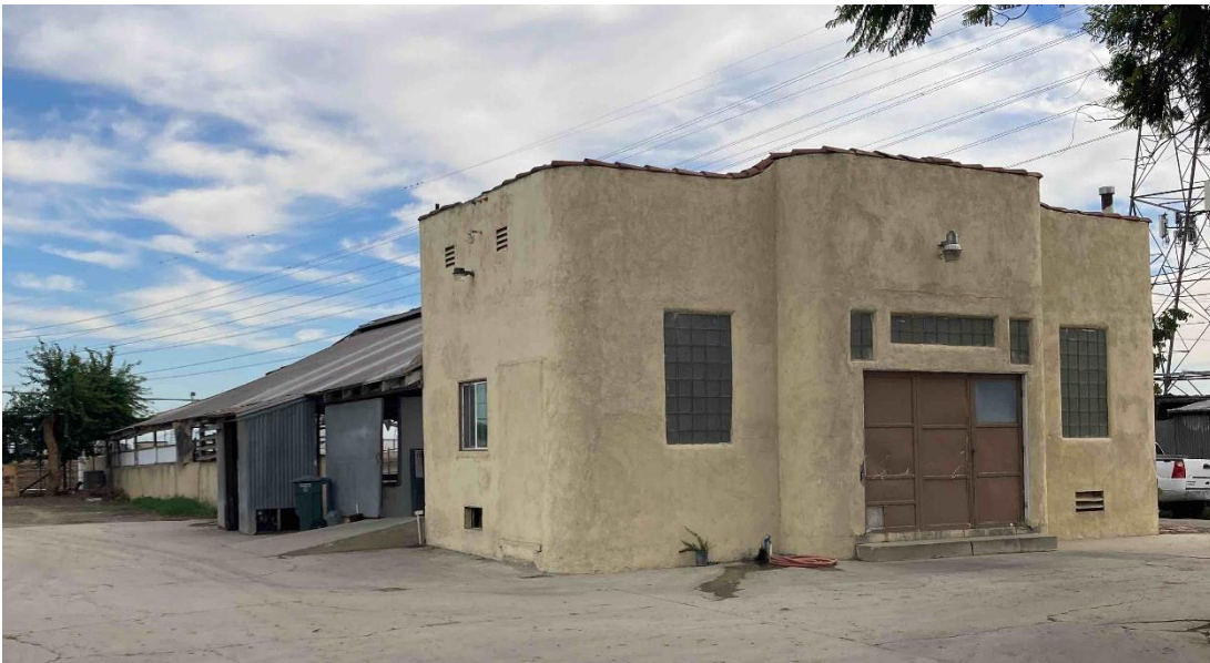
Photograph 7: 13813 Euclid Ave milk parlor, north and west elevations, camera facing southeast, October 31, 2022.
