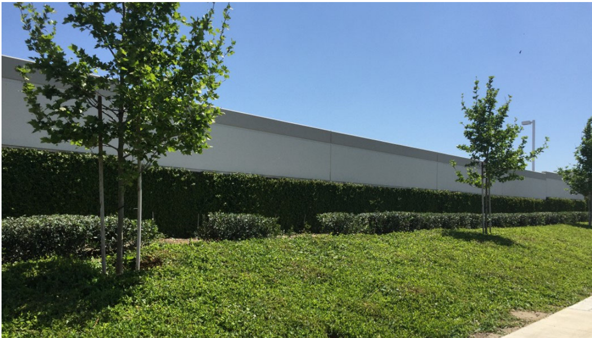
Photo 7.4-Example of typical screen wall with landscaping
