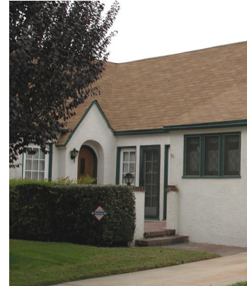
Recessed entry door with multi-paned windows and decorative light fixtures.
