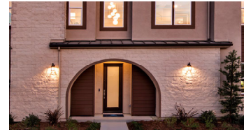
Entry porch with door on accent wall
