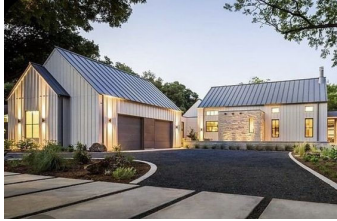
Simple roof forms with standing seam metal roof.
