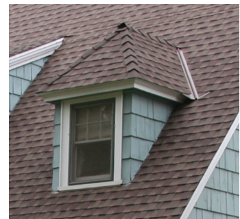
Multi-paned window in hipped dormer, extensive use of shingle siding.
