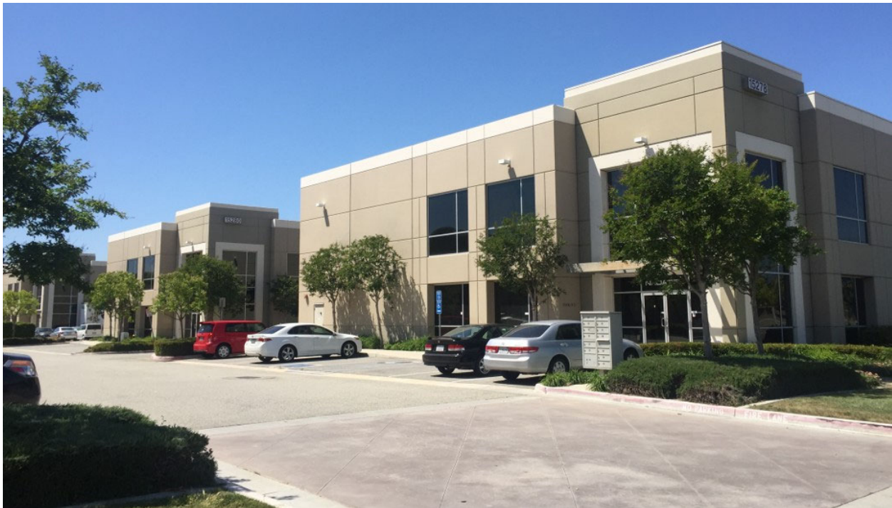
Photo 7.1 - Example of main building accents oriented towards street and entry
