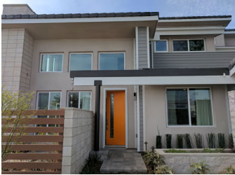
Low pitched roof with overhang and windows and doors flush with exterior wall.
