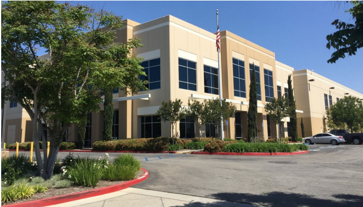
Photo 7.2 - Example of an Industrial edge along a perimeter street such as Hamner Avenue
