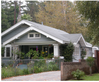
Low slope gabled roofs with large overhangs.
