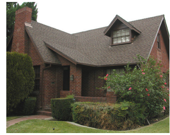
Covered Front porch with extensive use of brick veneer.
