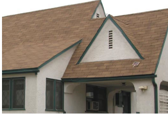
Steep roof pitches with articulated massing and gable end venting as accents.
