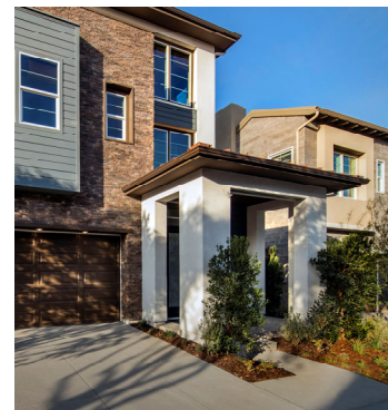
Covered entry porch with low-pitched roof
