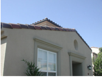
Low pitched gabled roof with simple recess at gable ends and cementitious window and door surrounds.
