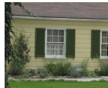
Simple repetitive windows with minimal treatment, can have shutters.
