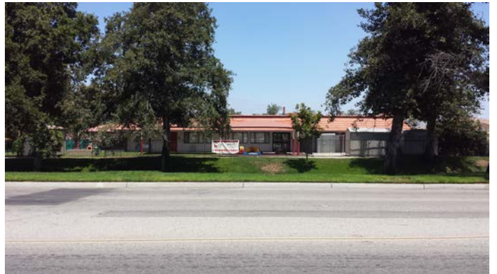
View of an adjoining property to the north
