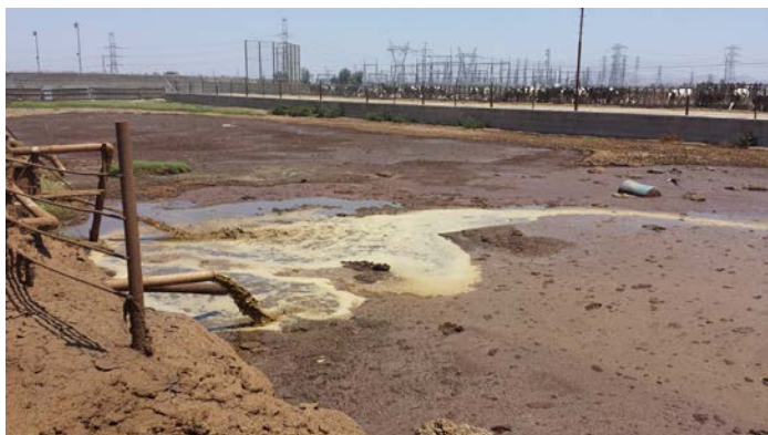
View of leaching pond on southern portion of the dairy
