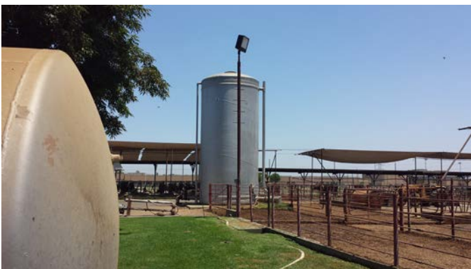
View of water tank
