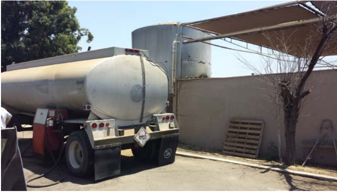
View of diesel fuel AST onsite
