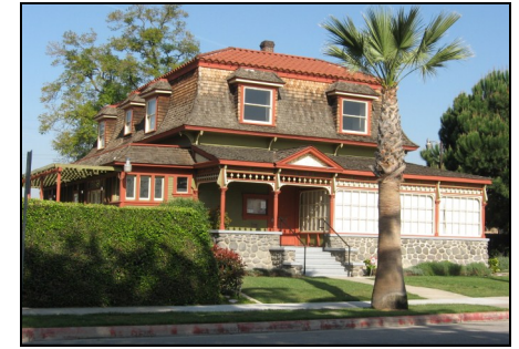
William Barton Fallis House~ Built 1892 Local Landmark No. 1
