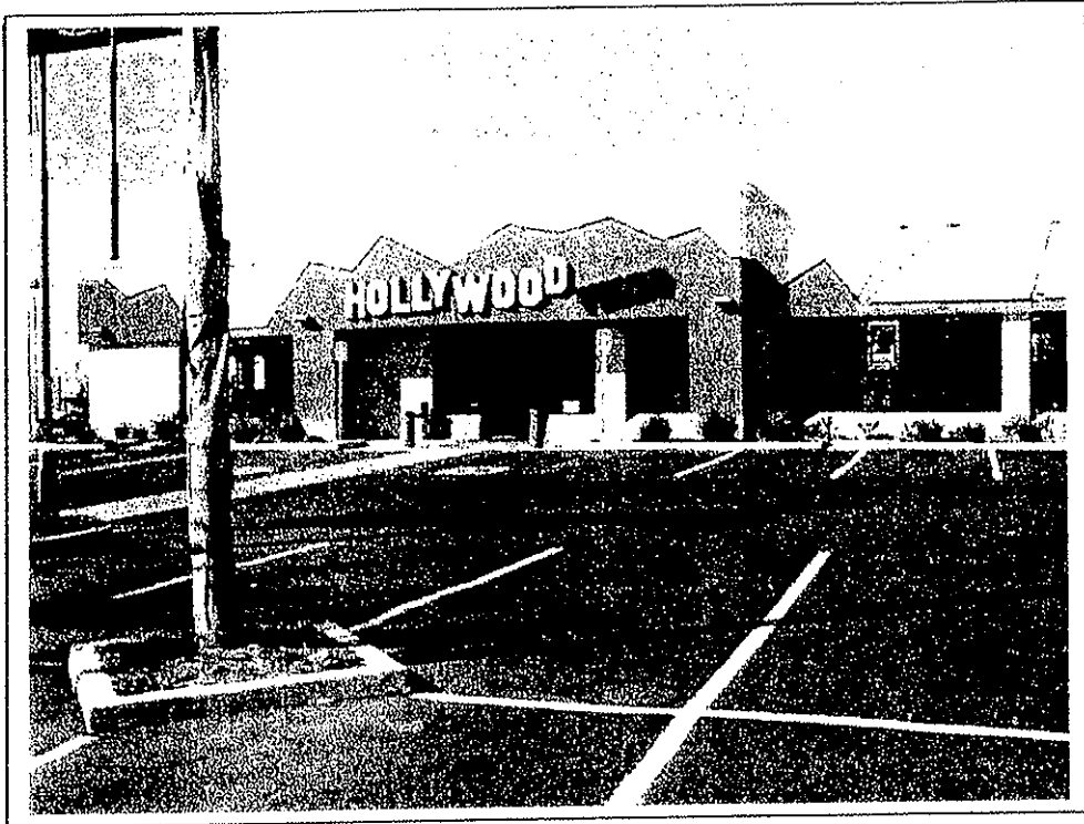
Photo 1. Northeastern portion of subject property, view looking west.
