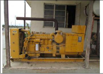
20. View of diesel-powered emergency generator and associated AST (size about 50-gallons) located outside milking-operations building at subject property. No AST leakage or staining of concrete observed.
