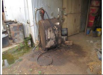
27. View of small AST (less than 100-gallons) containing oil with stained soil surrounding.
