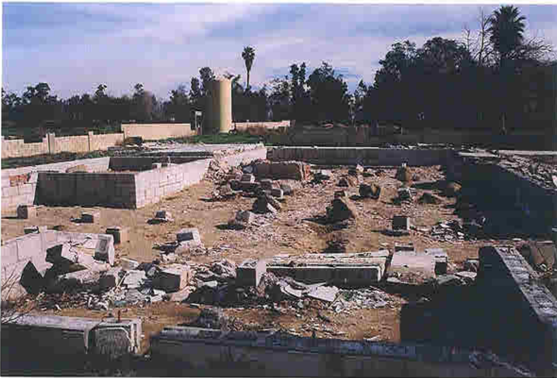
Photo 4 - Residential foundation (1 of 2) and water tank located on north side of Eucalyptus Ave.
