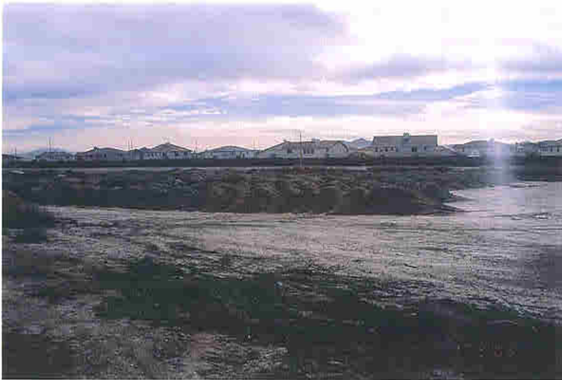
Photo 14 - Typical view of fill material that covers 1/3±rd of the southern 1/3rd of the site.
