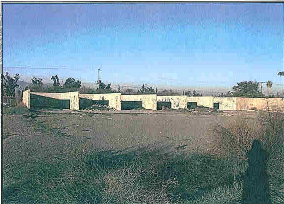
Former storage areas (concrete and block), south of Eucalyptus Avenue, east of Cleveland Avenue.
