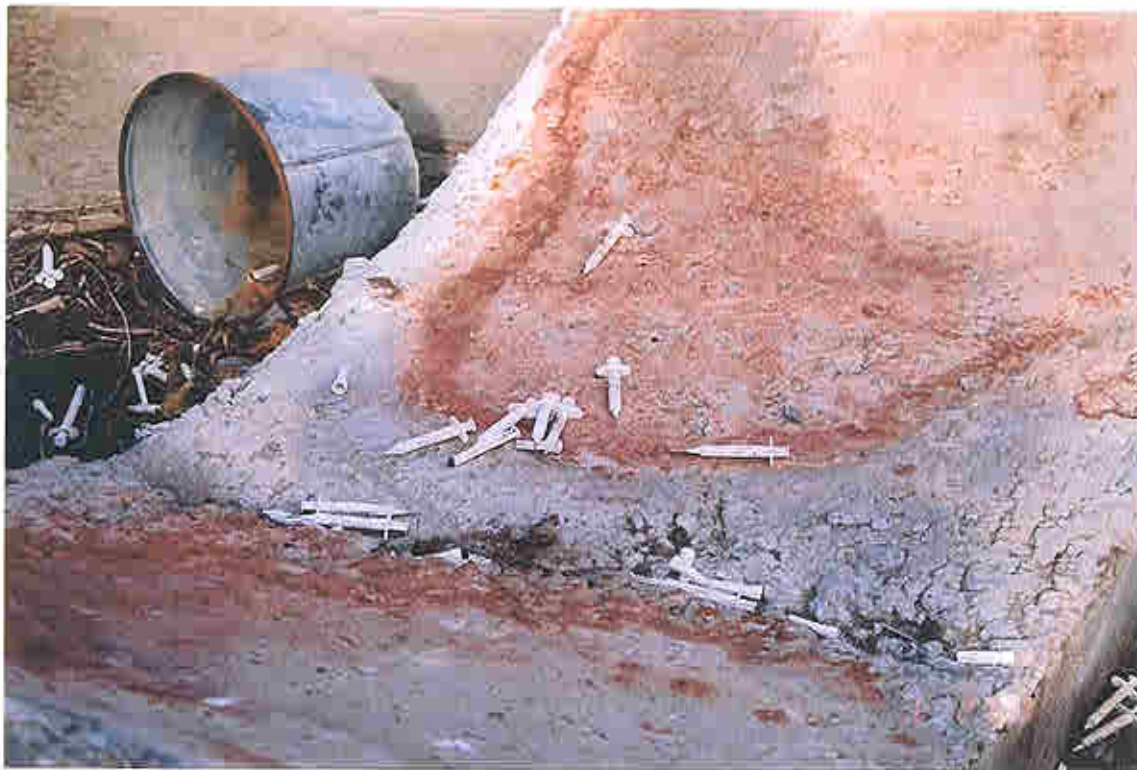
Photo 10 - Syringes within abandoned concrete cradle for above ground fuel tanks. Possibly used during dairy operations.
