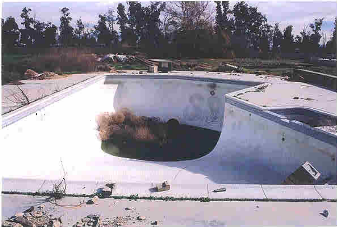
Photo 5 - Residential swimming pool located on north side of Eucalyptus Ave.
