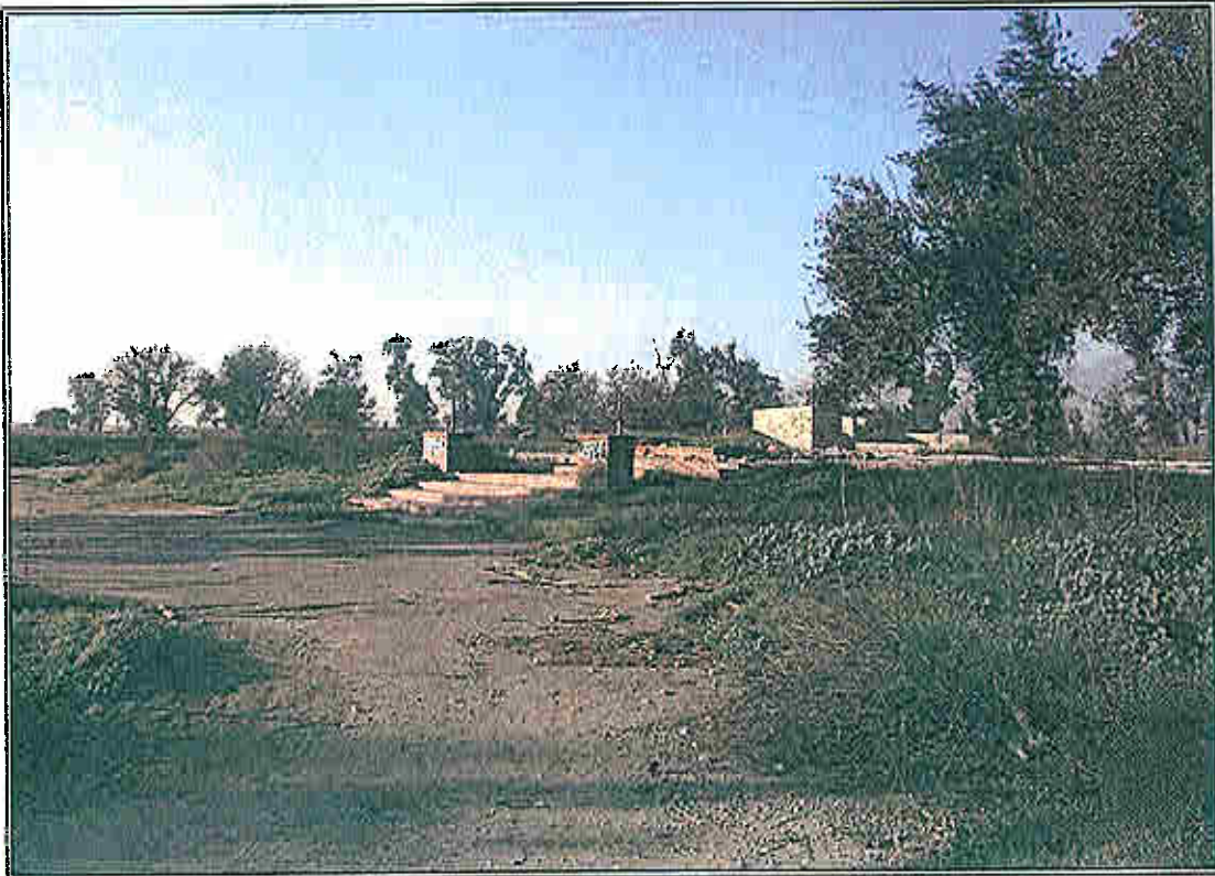
Concrete foundation and asphalt drive on the northern property.
