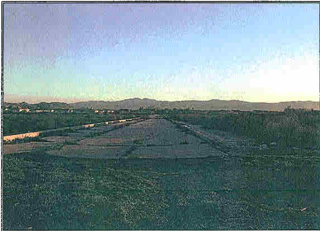
Concrete foundation (former dairy) on the southeast side of the site.
