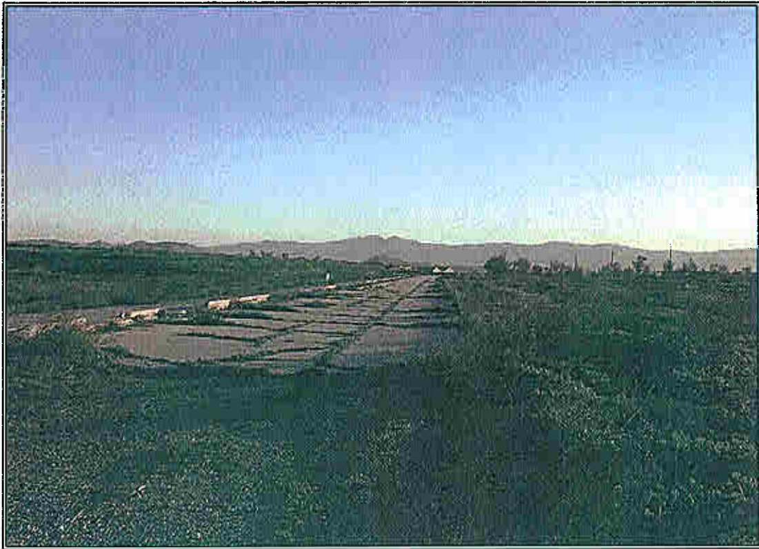
Looking south along concrete foundation (former dairy), southwest side of the site.
