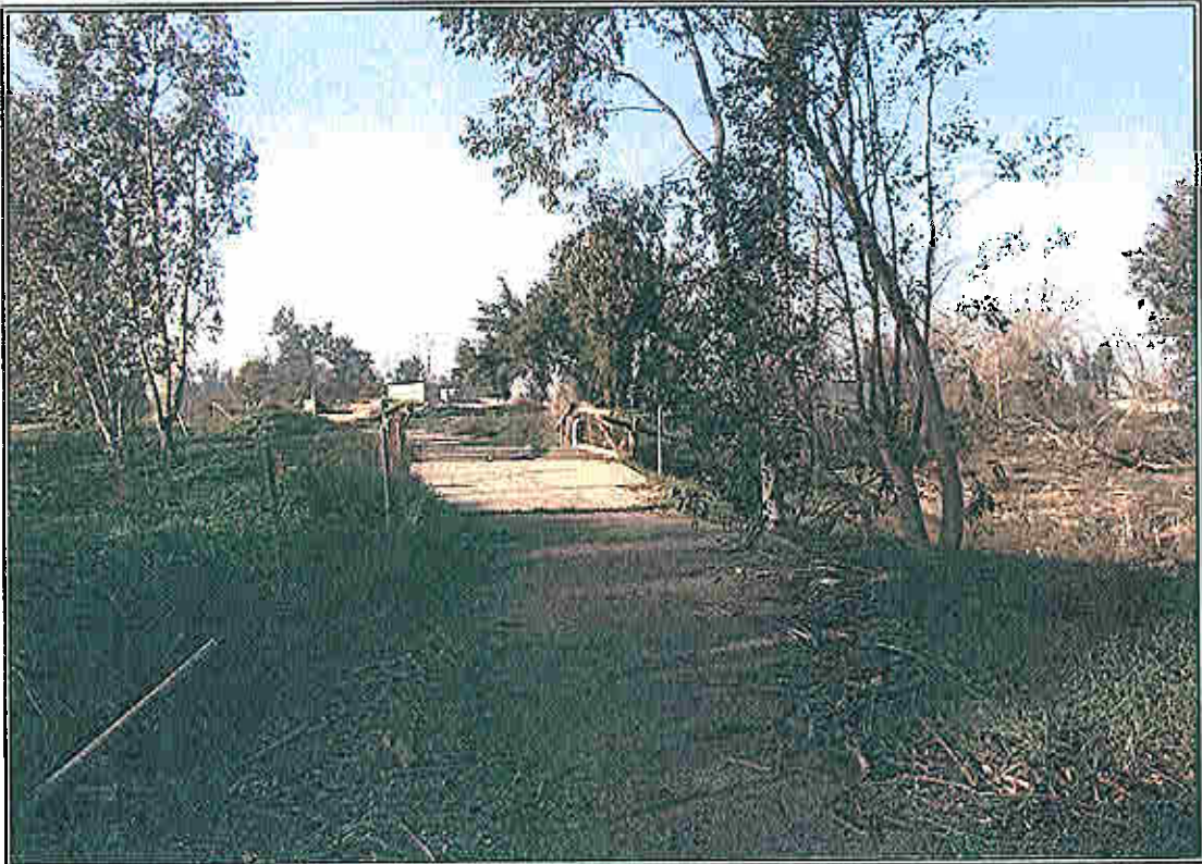
Asphalt and concrete drive with wood bridge over empty pond area.
