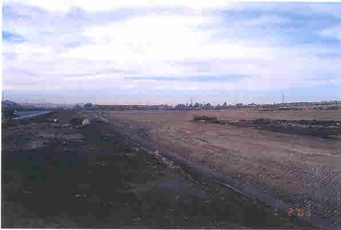
Photo 2 - View of earthen basin constructed at the southwestern corner of site.
