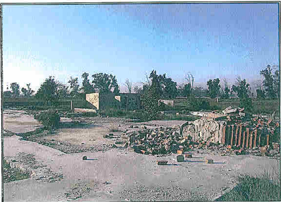
Concrete foundation, birch fireplace and block structure.
