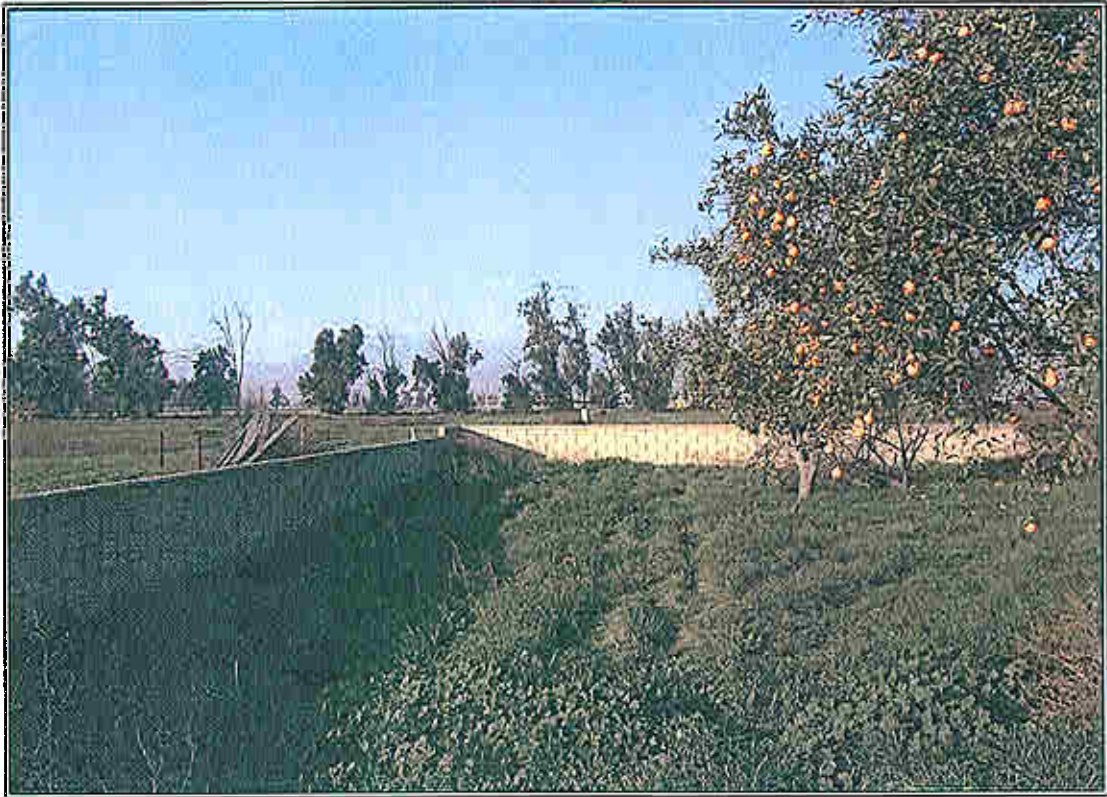
Block wall, and standing concrete pipe.
