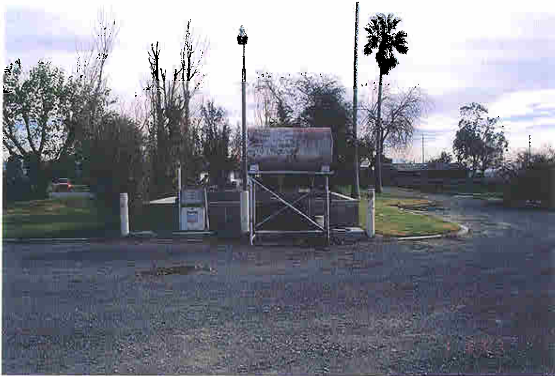
Photo 9 - Above ground fuel tank, fuel pumps (dismantled) and concrete cradle for above ground fuel tanks.
