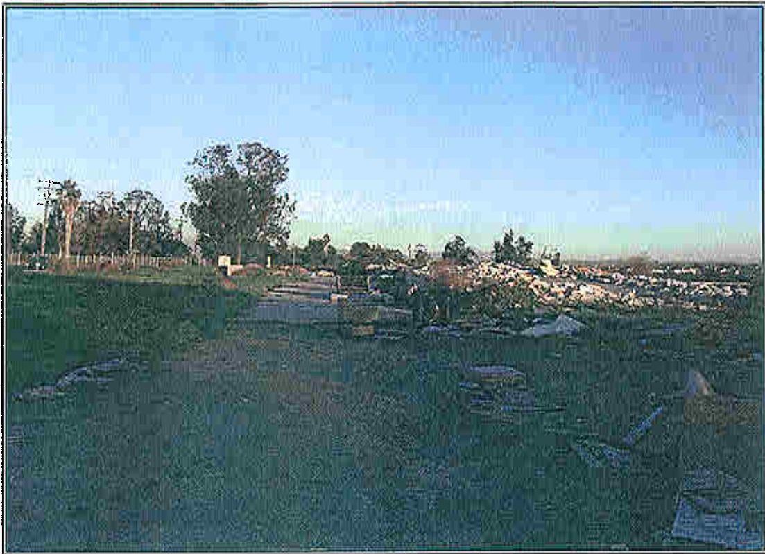
Looking east at debris and former dairy foundation near the center of the site.
