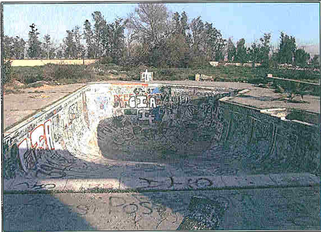
Concrete pool near former residence on north portion of the site.
