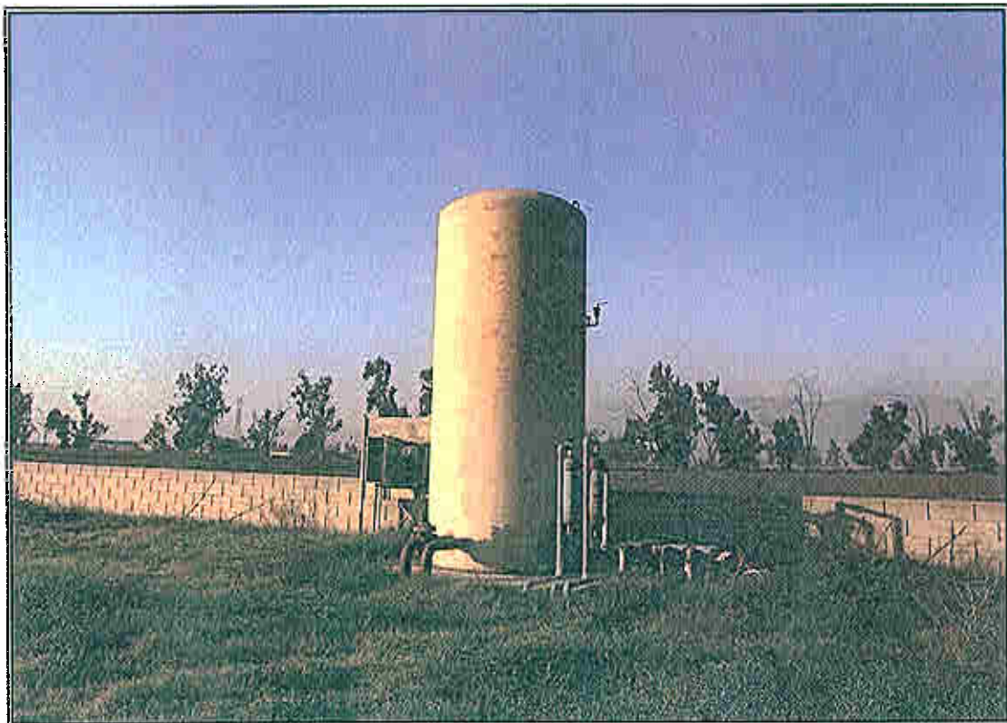
Approximately 5,000 gallon water tank near block wall on northern property.
