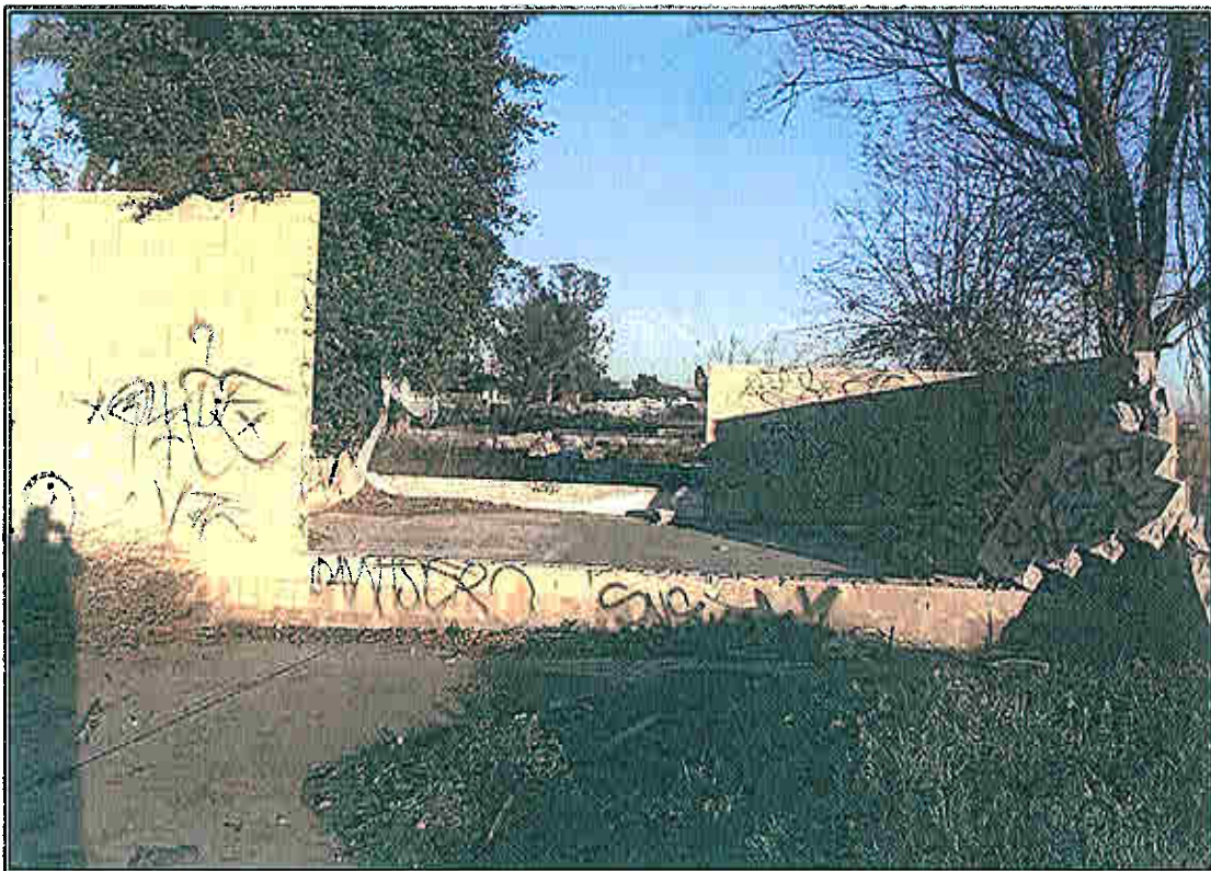
Looking east at concrete and block wall, south of Eucalyptus Avenue.
