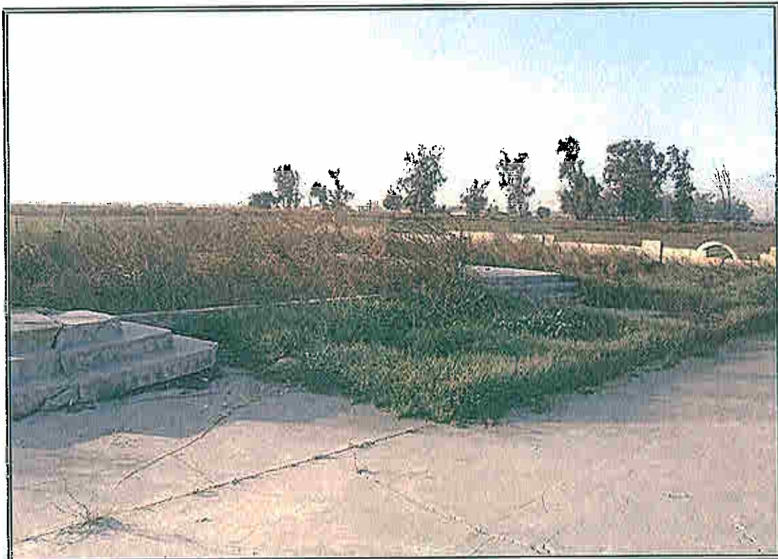
Concrete foundation (former residence) on the northern property.
