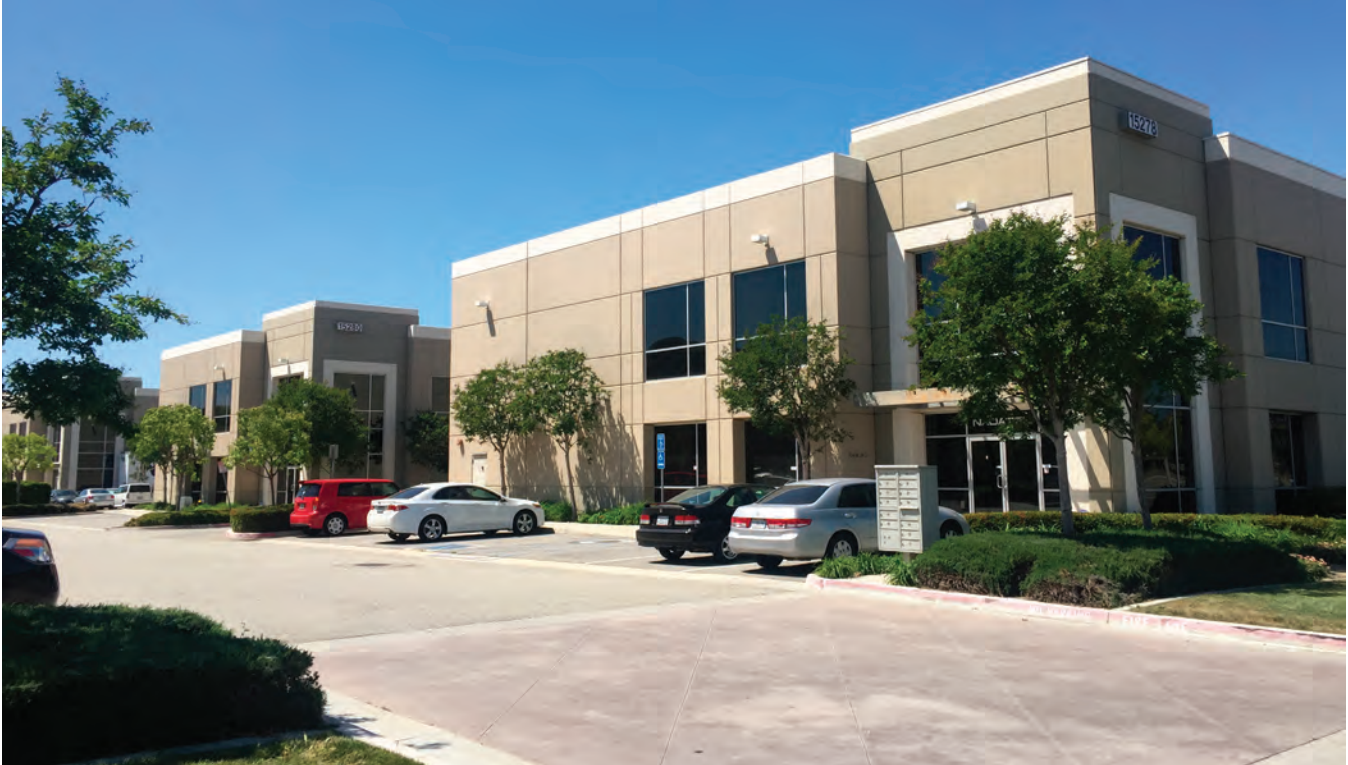
Photo 7.2 - Example of smaller scale business/industrial park buildings
