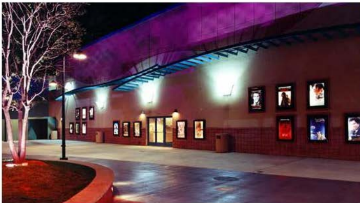
Figure 3: Exterior of the AMC Ontario Mills 30 Theater
