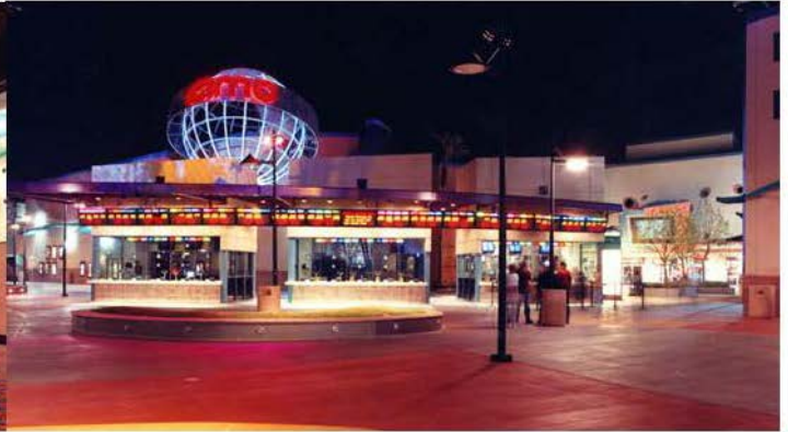
Figure 2: Exterior of the AMC Ontario Mills 30 Theater
