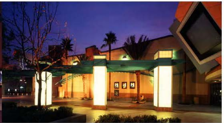
Figure 4: Exterior of the AMC Ontario Mills 30 Theater
