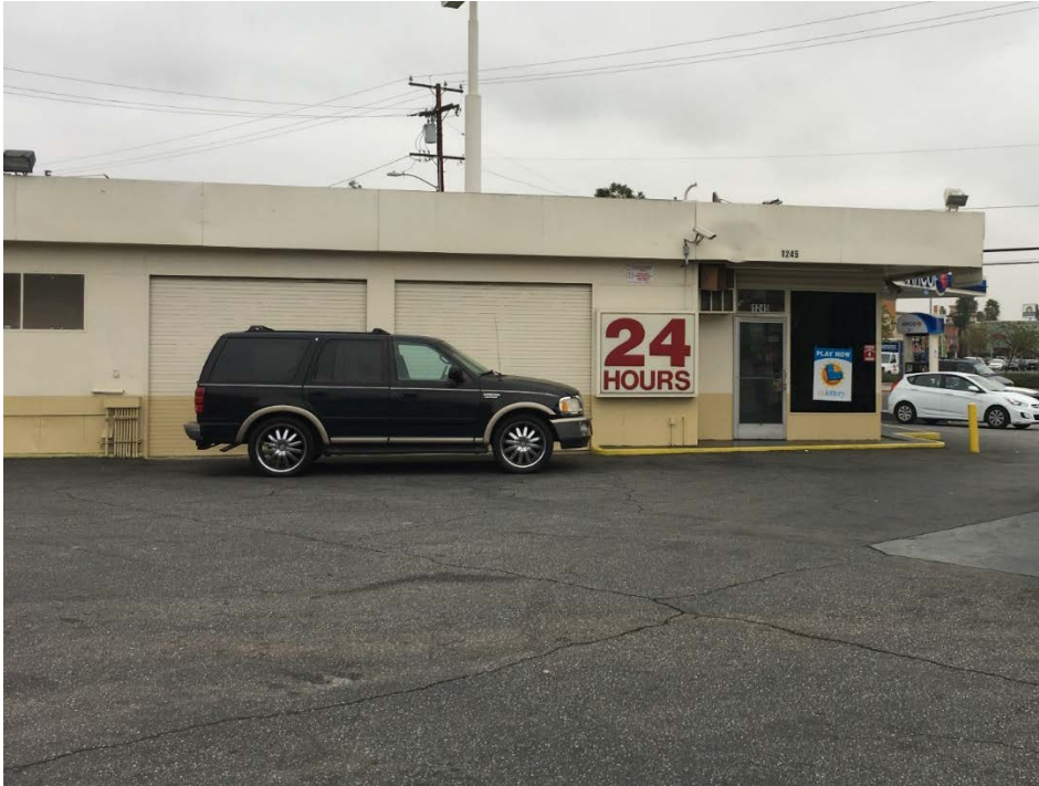
Southwest elevation: garage bay doors, cabinet sign to be removed
