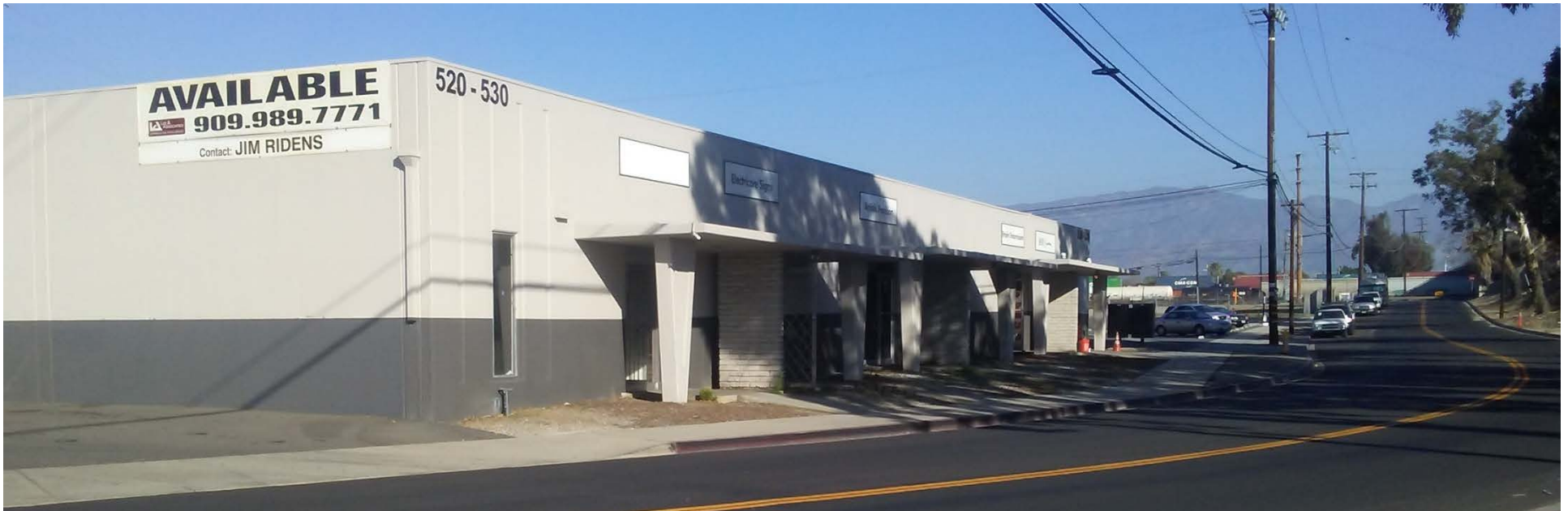
SOUTHEAST VIEW OF EXISTING INDUSTRIAL BUILDING
