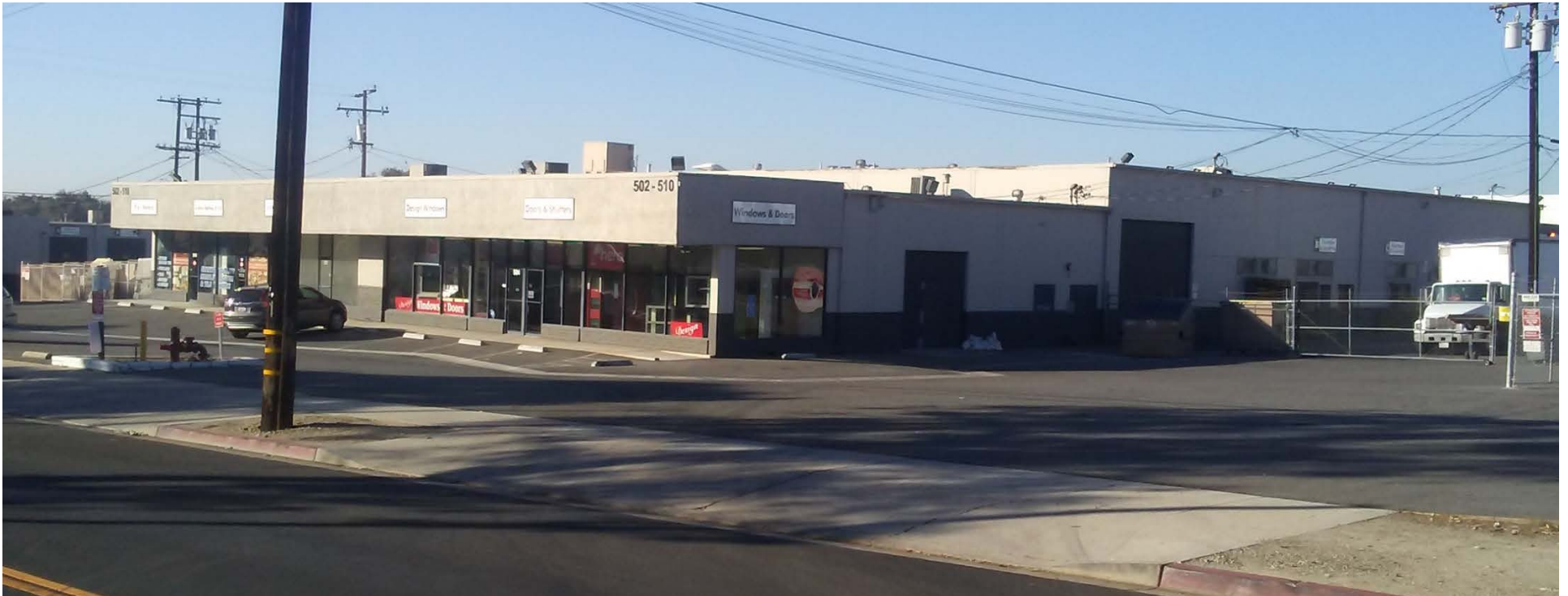
NORTH VIEW OF EXISTING INDUSTRIAL BUILDING
