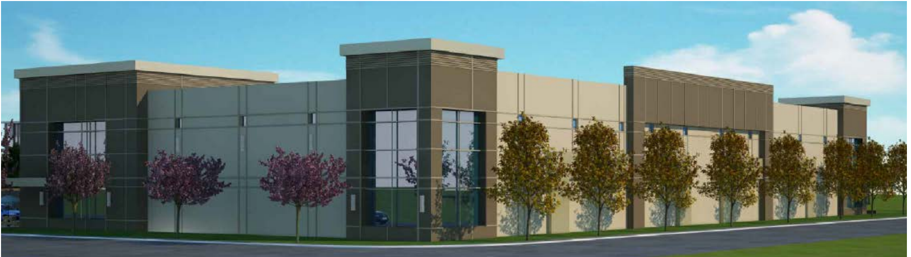
View of Northwest Corner of State Street & Mountain Access Road
