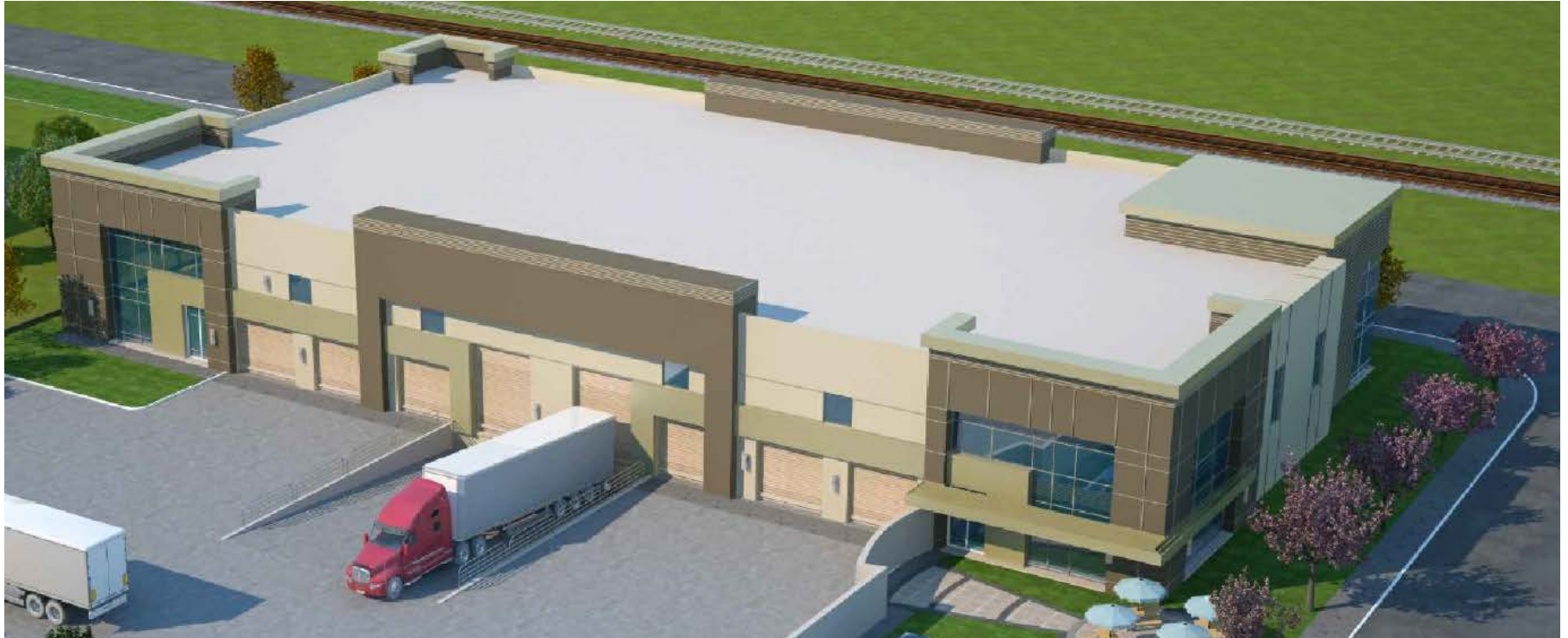
Southeast View of Building from Mountain Avenue Bridge
