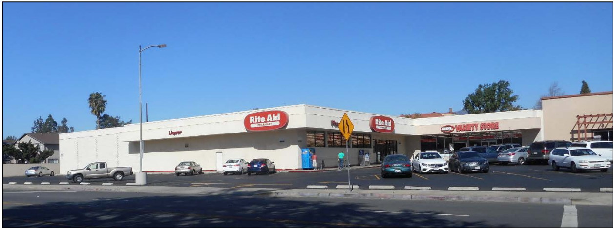
Adjacent Commercial – View looking northwest from G Street
