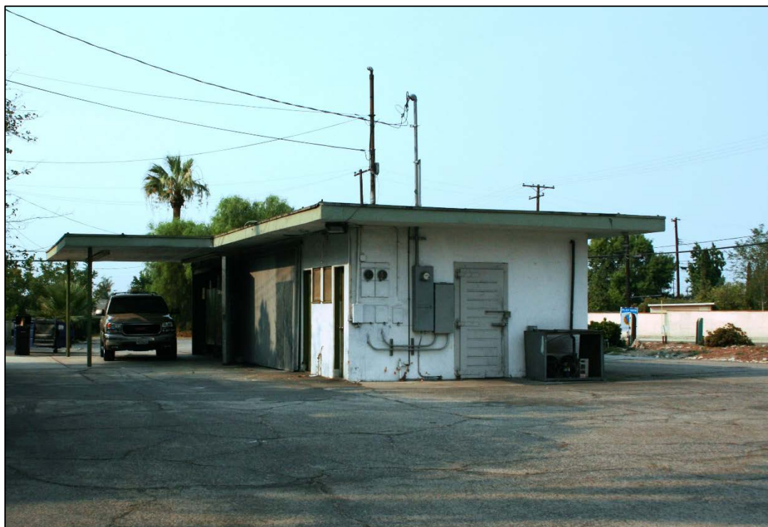
Convenience market, view looking southwest
