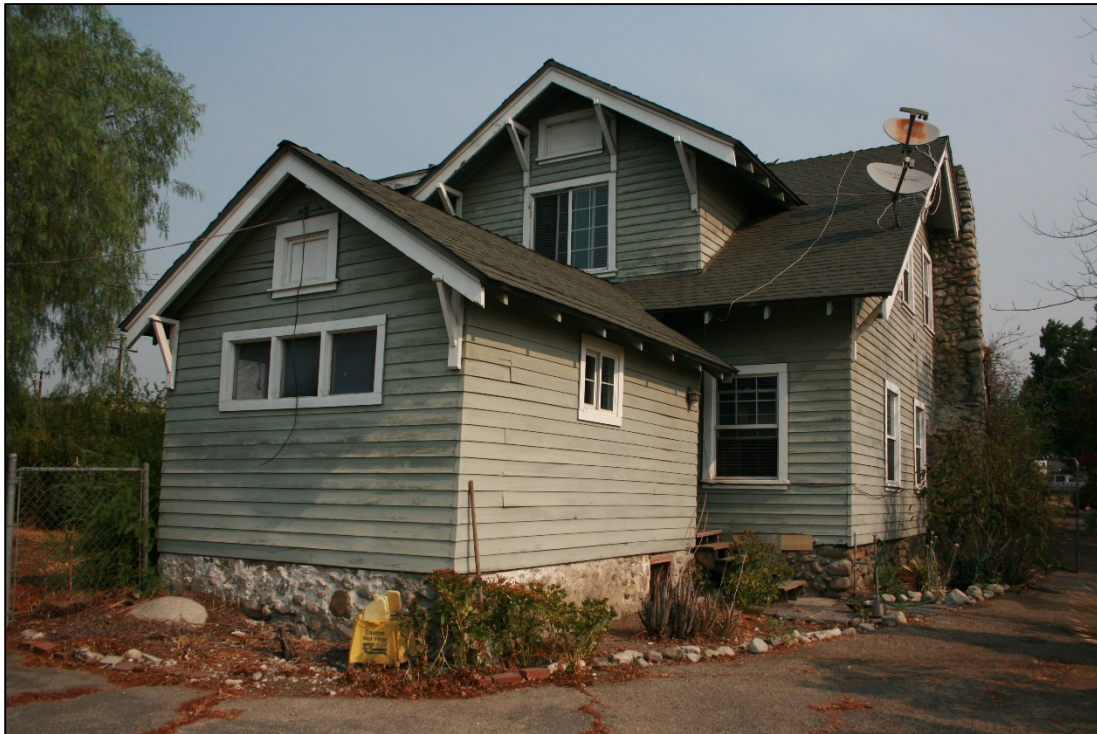
Rear addition, view looking northwest
