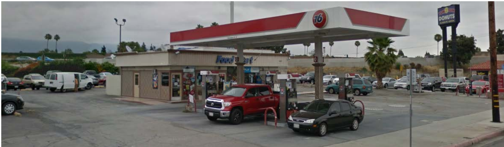
Southeast View of Existing Canopy
