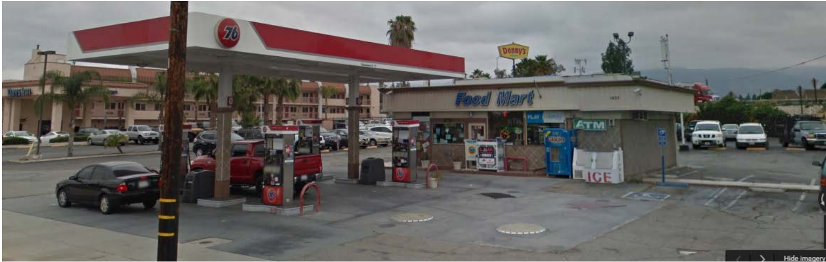
Northwest View of Existing Canopy
