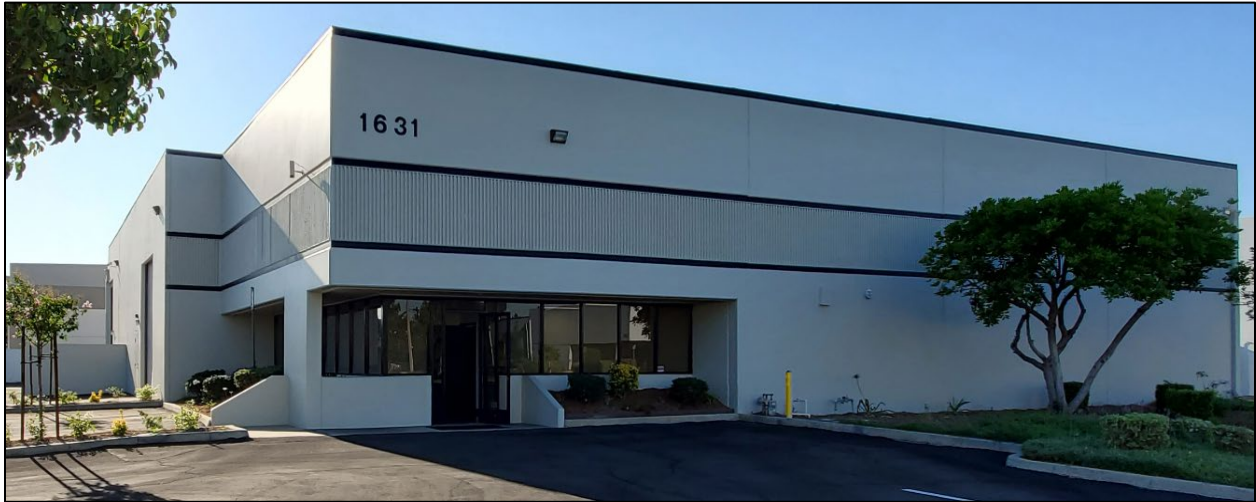
Northwest Corner View of Building
