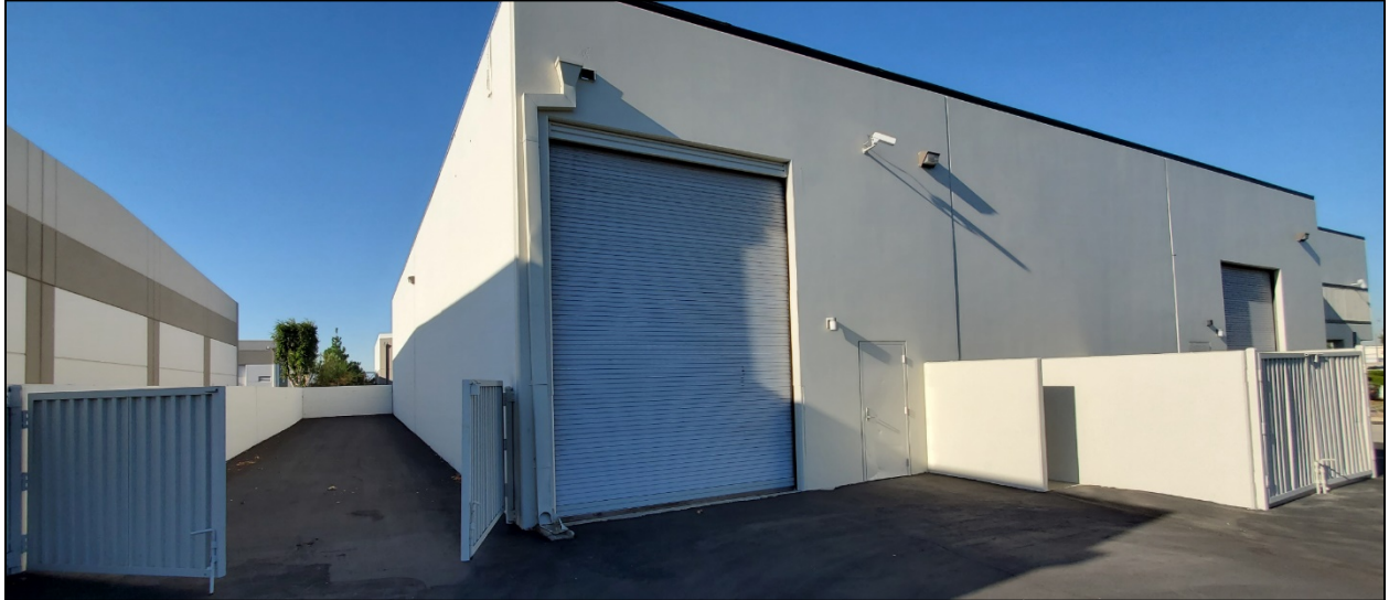
Northeast Corner View of Building
