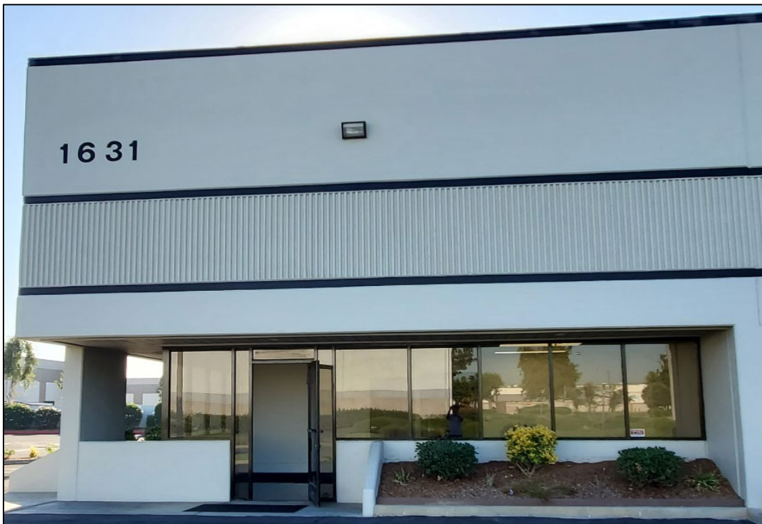
Building Main Entrance: West Side View from Parking Lot
