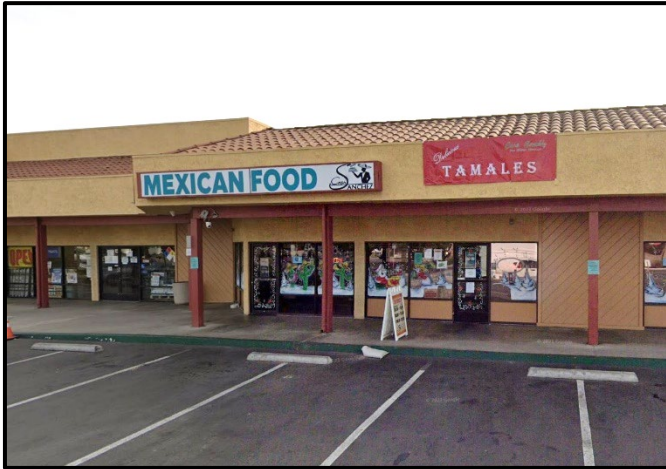
Figure 1: Street View of Project Site
