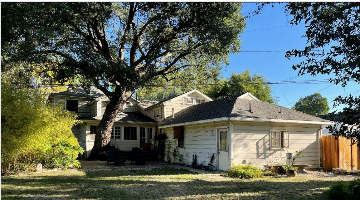
Avenue Boarding House - View looking northeast
