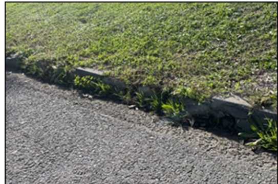
Figure 2: Buried Rock Curb
