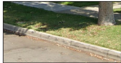
Figure 3: Scored Concrete Curb
