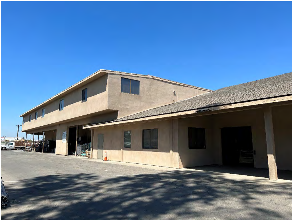
G-2. View of the western portion of the main building, office space and warehouse storage (8/29/2022).
