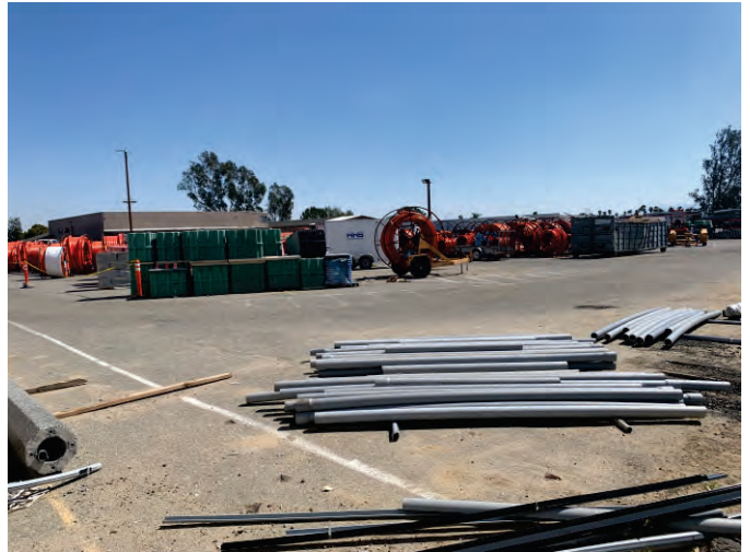
4. View of general site conditions.
