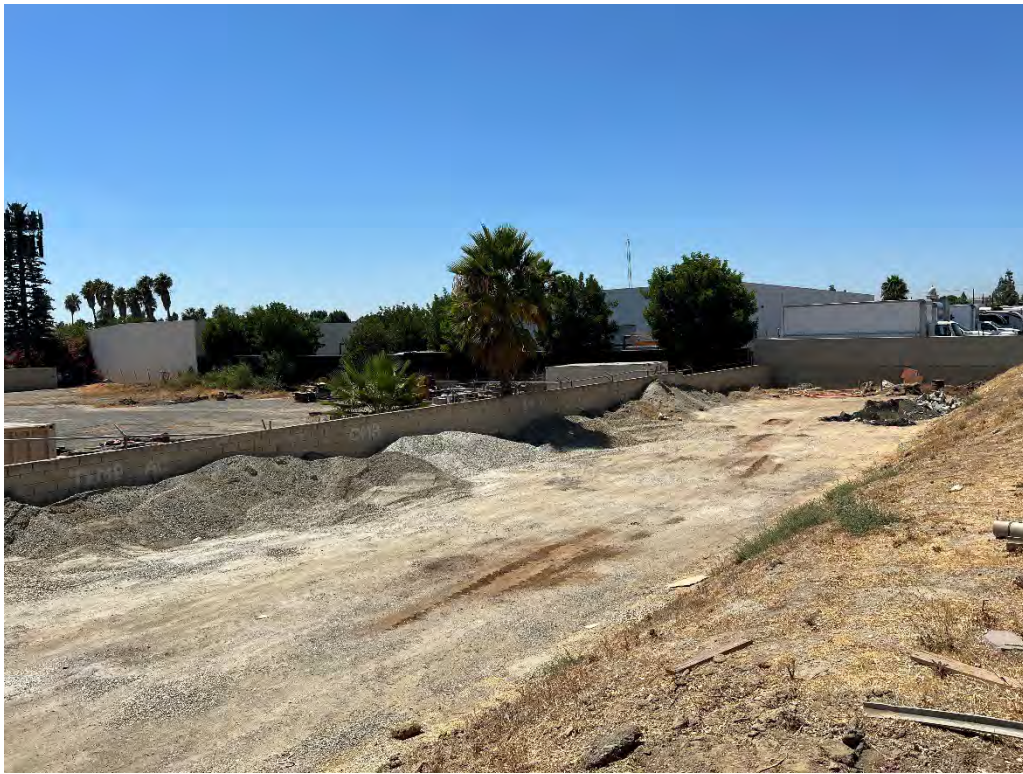
G-15. Construction material, asphalt, and gravel, staged along the southern boundary (8/29/2022).
