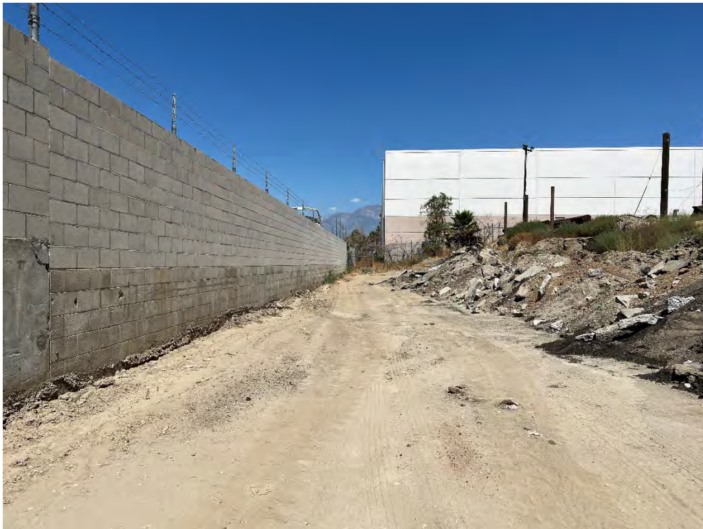
G-16. Material generated off-site from excavation/trenching staged along the western boundary (8/29/2022).
