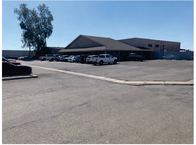
2. View of general site conditions.
