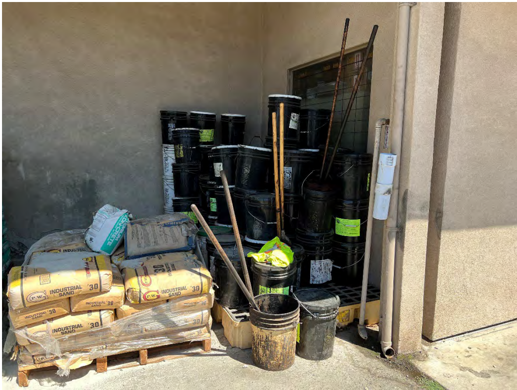
G-3. Sealant and emulsion products stored off ground behind the main building (8/29/2022).
