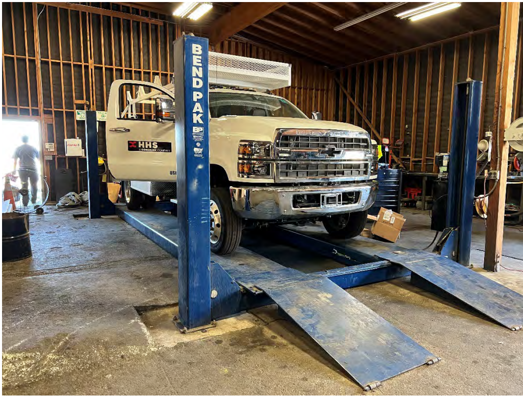
G-7. Aboveground hydraulic lift in the secondary building (8/29/2022).
