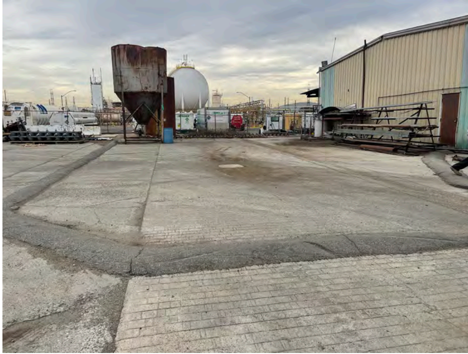
Photograph 3: Bermed truck-washing area by Building B.
