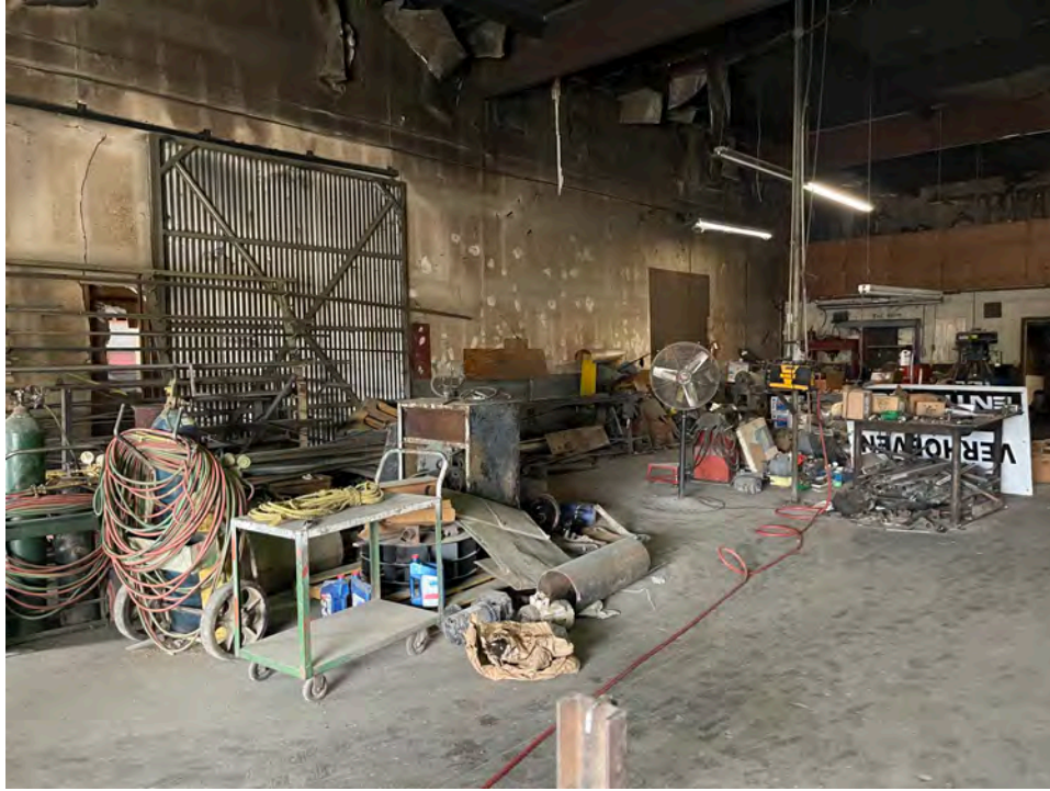
Photograph 15: Verhoeven equipment service area in Building A.
