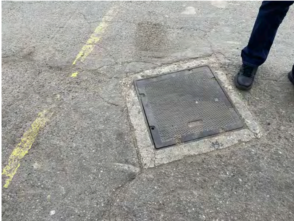
Photograph 11: Septic tank location by Building A.
