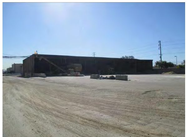
Photo #6 View of the storage shed located on the central portion of the site.
