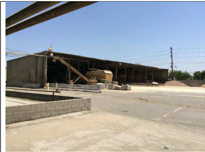
9. View of Grain Storage (Building E)
