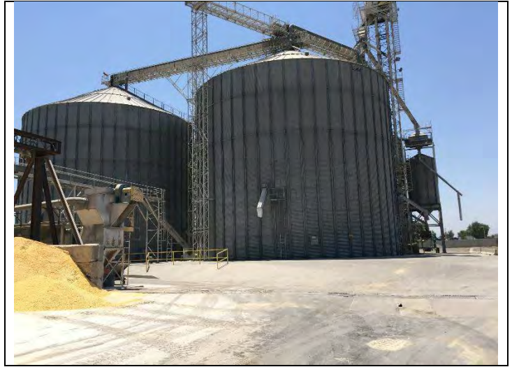
8. View of Storage Silos
