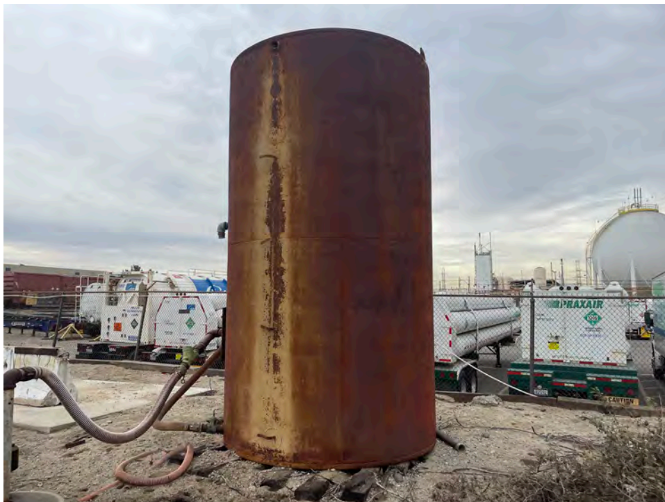
Photograph 2: Wash water storage tank by truck-washing area.
