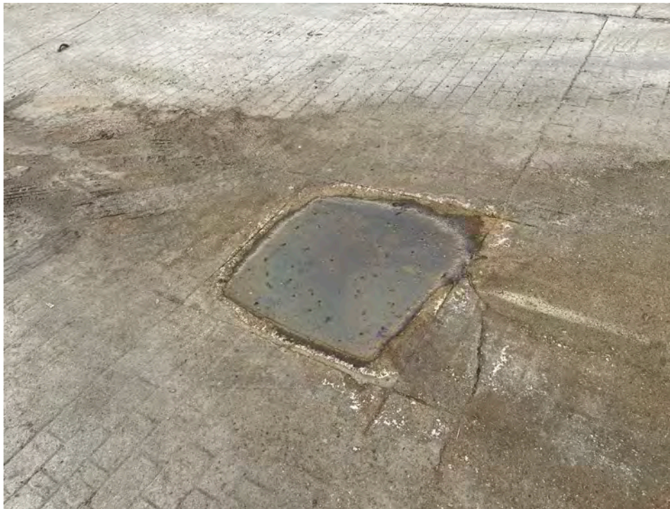
Photograph 4: Sump in truck-washing area.
