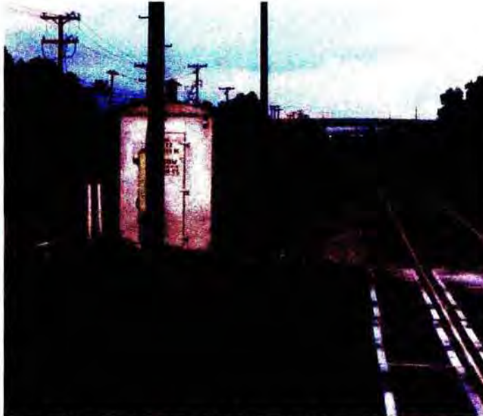
San Pedro, Los Angeles and Salt Lake Railroad at Monte Vista Avenue. Alignment looking west from Monte Vista Avenue with call in booth. November, 2012.
