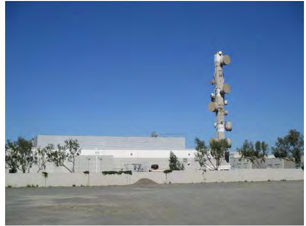
Photo #28 View of Verizon Wireless located to the adjacent west of the site.
