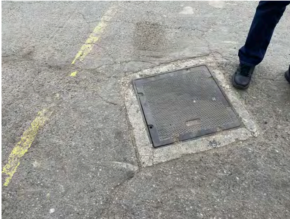
Photograph 11: Septic tank location by Building A.
