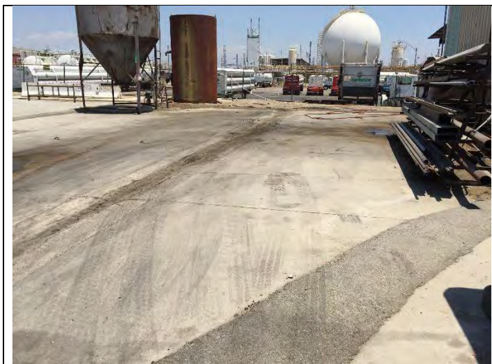
14. View of Former Vehicle Wash-Down Area
