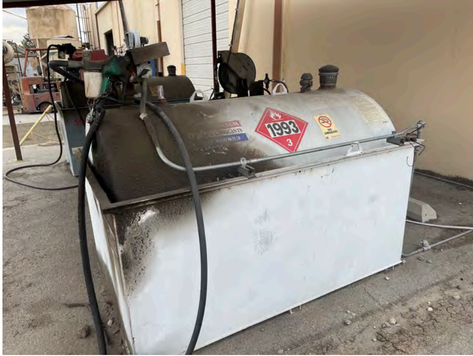
Photograph 5: Diesel fueling area by Building A.
