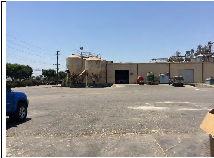
3. View of Main Building (Building A)
