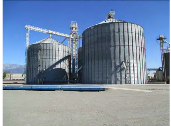
Photo #2 View of the large storage silos located on the western portion of the site.
