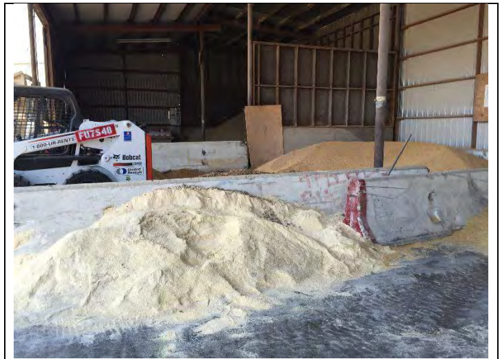
10. View of Grain Storage (Building D)
