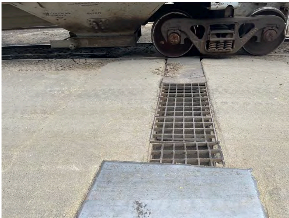
Photograph 12: Rail transloading area.
