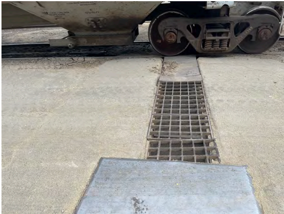
Photograph 12: Rail transloading area.
