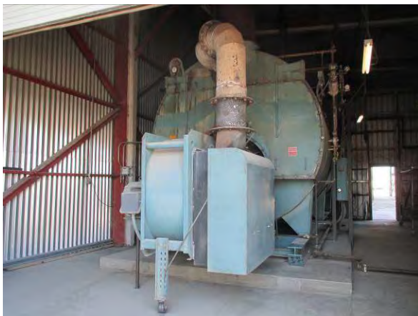
Photo #11 Typical interior view of the boiler area.
