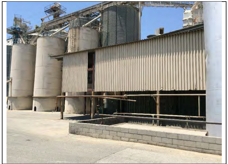
4. View of Milling Area
