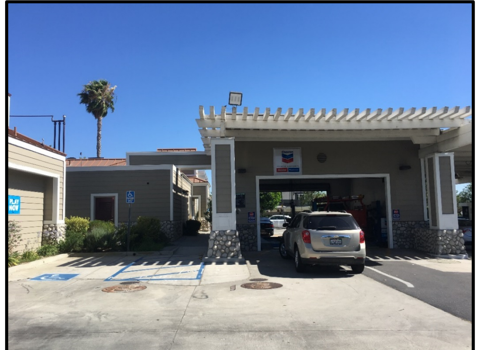
View looking south at existing convenience store (to remain) and oil service bay (to be removed)
