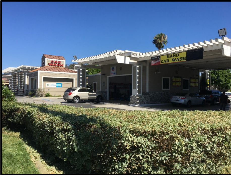
View looking southwest at existing oil service bay to be removed
