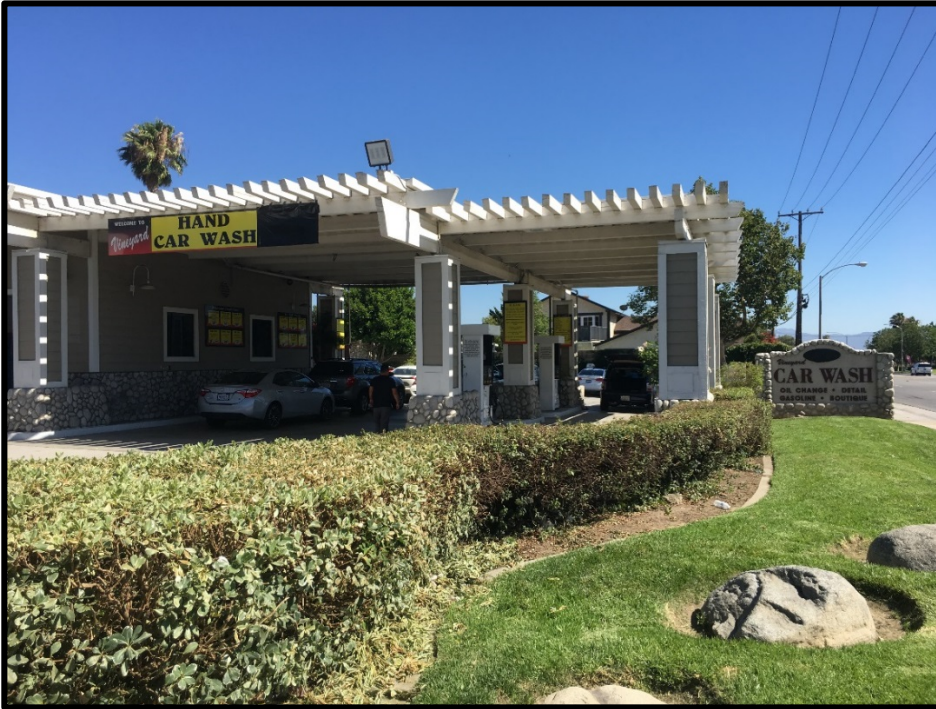
View looking southwest at existing fuel station to be expanded
