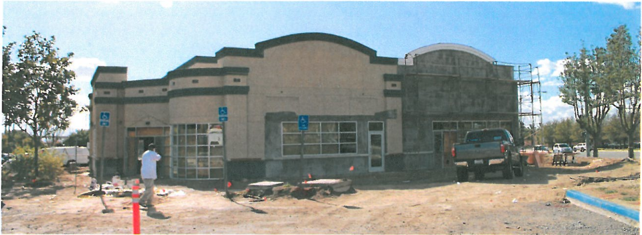
Above: project site currently under construction
