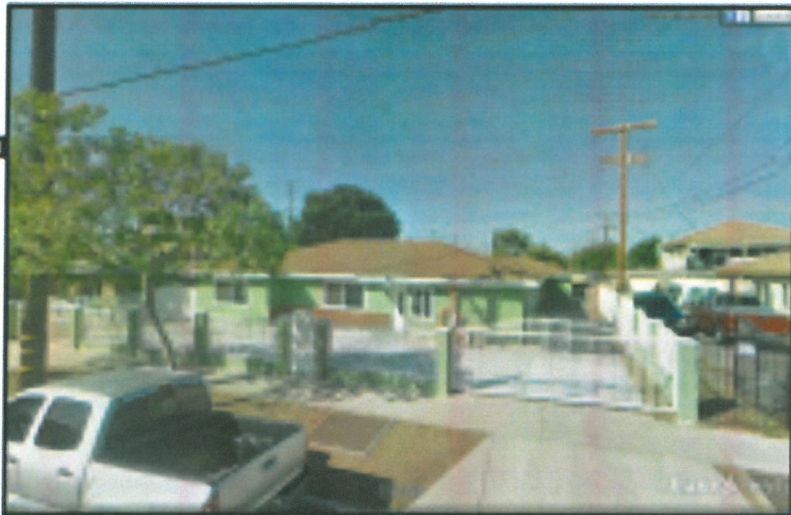
1118 South Campus Avenue – Existing Building
