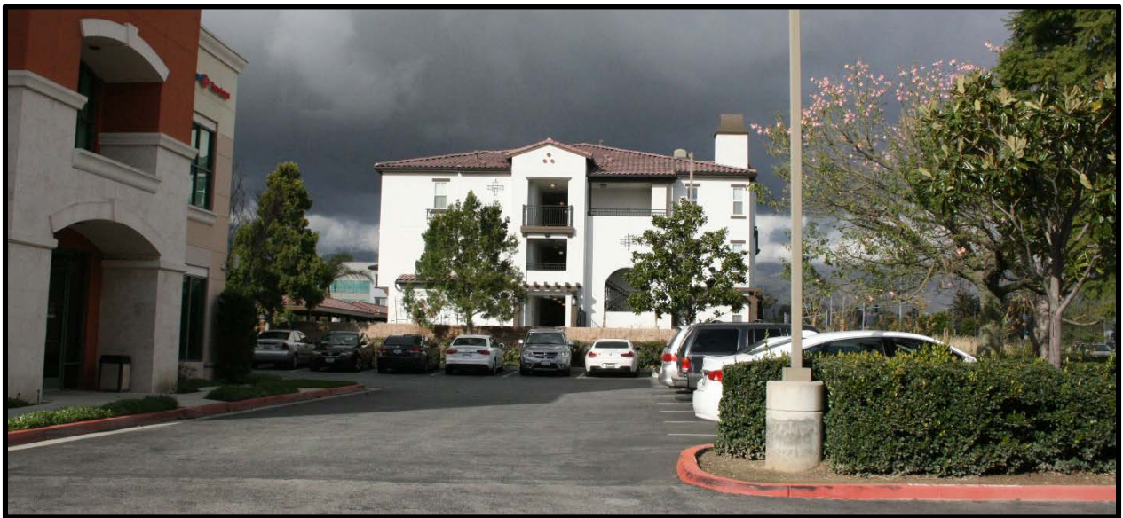
View looking north at existing multi-family buildings
