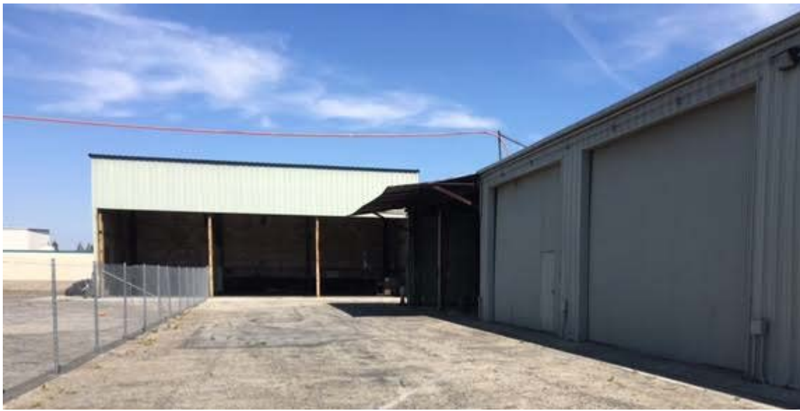
Existing Shop Building at Rear of Main Building – Looking East from Campus Ave
