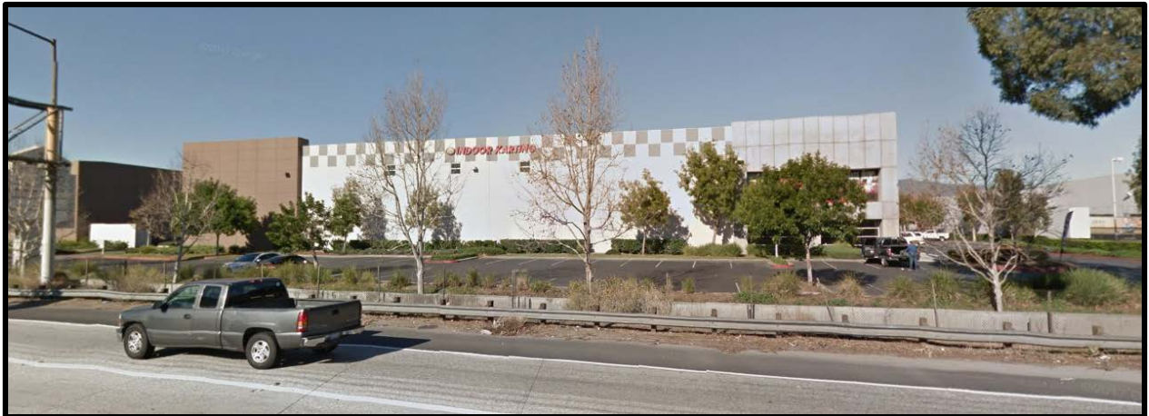
View looking south at project site from I-10 Freeway
