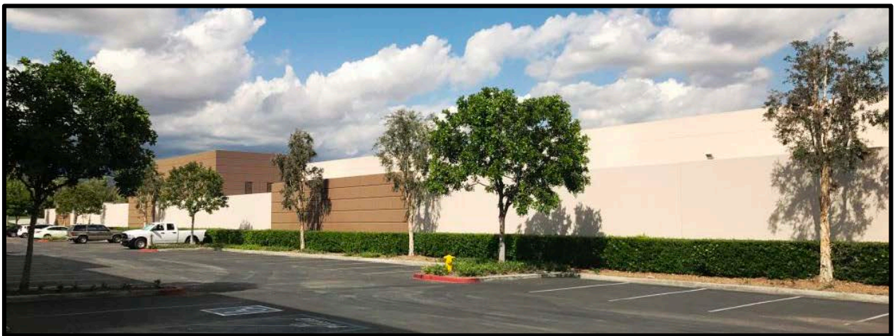
View looking west at neighboring industrial building
