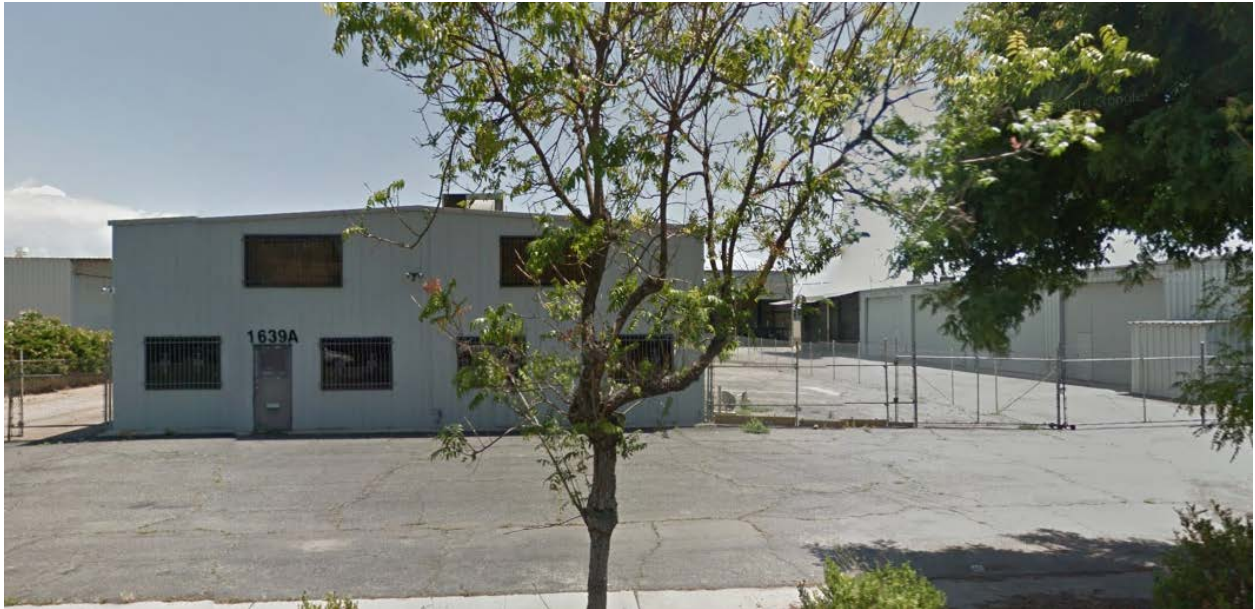
1639 S. Campus Avenue, Unit A – View Looking East from Campus Avenue
