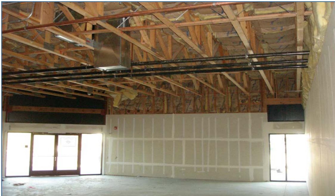
Existing interior condition of future BaronHR space
