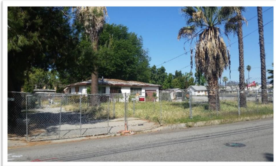
Southern Portion of Site- Looking North on Magnolia Avenue
